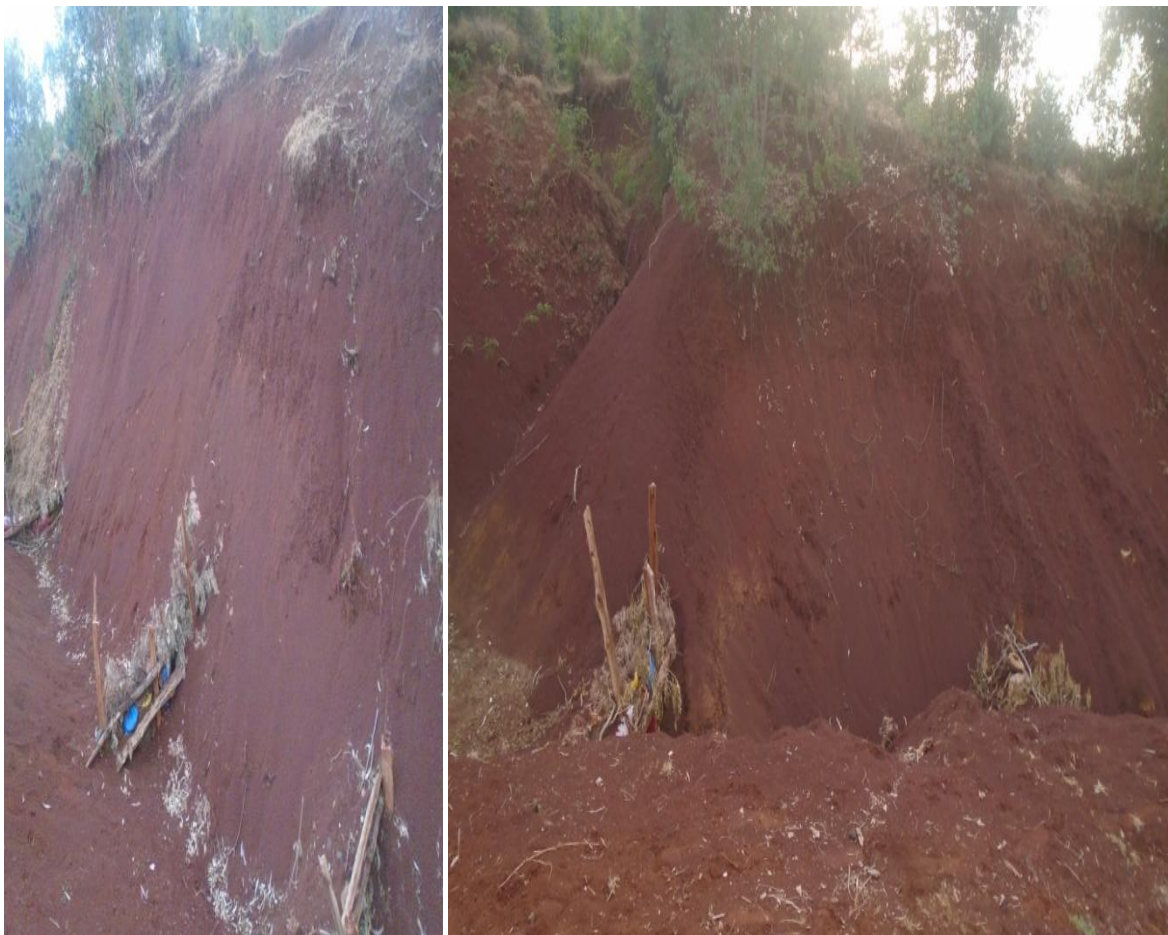
Plate 1 Gully erosion near the catchment area
