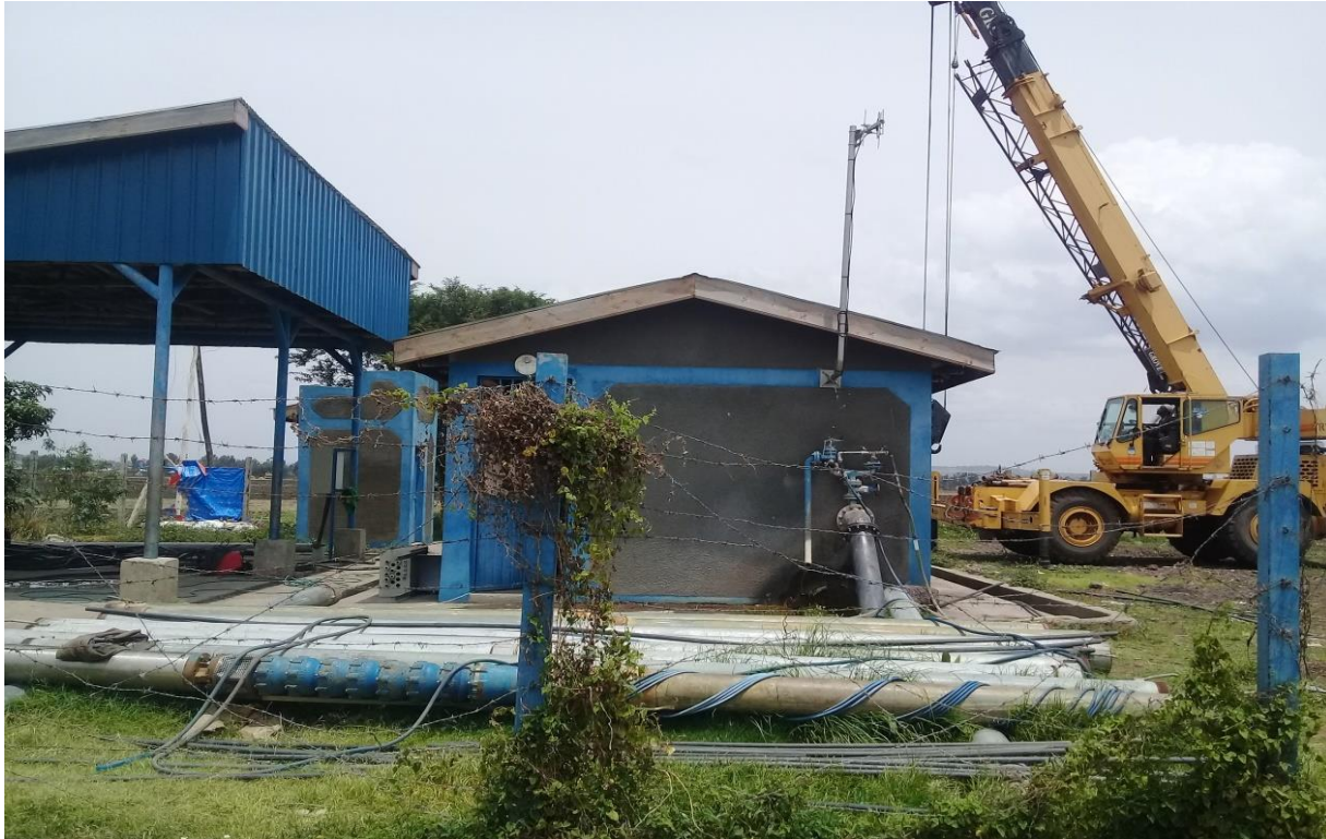
Figure 18:- : Borehole WF01-PW14 under maintenance
