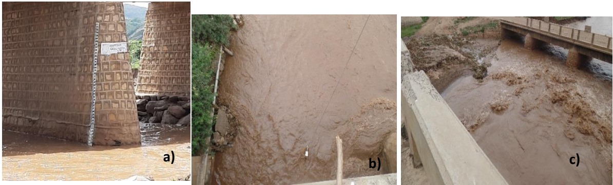
Figure 7.2. Upper Erer River at Bridge: a) Staff gauge reading re-installed (2020), (b) Flow measuring process on site using crane movement for vertical current meter (2020) and c) Rivers at full stage during peak flow (August 2020).
