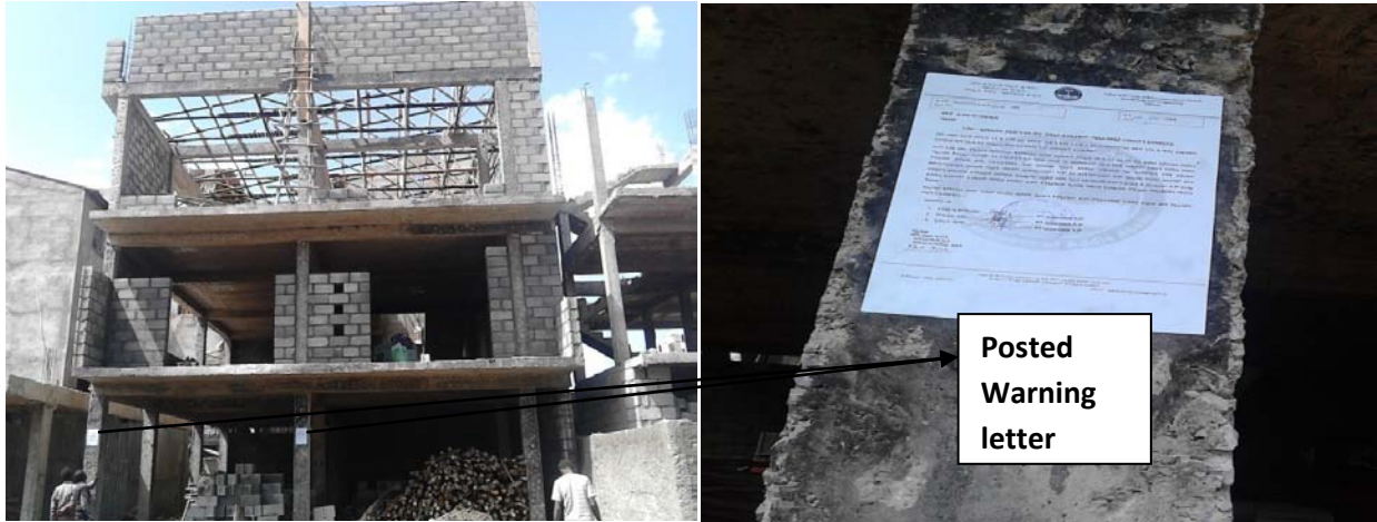
Photograph 4.4: House construction made on the plot of terminated lease agreement
