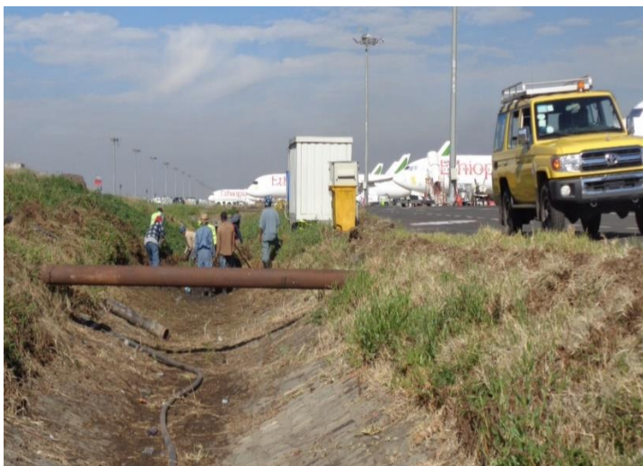
Water way management (December 2019; Photo: Fekadu Assefa)
