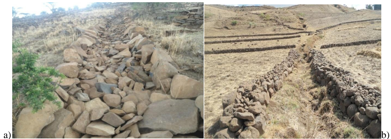
Fig5.5:- Stone water way (a) and traditional grass waterway (b) (Field survey, 2014)
