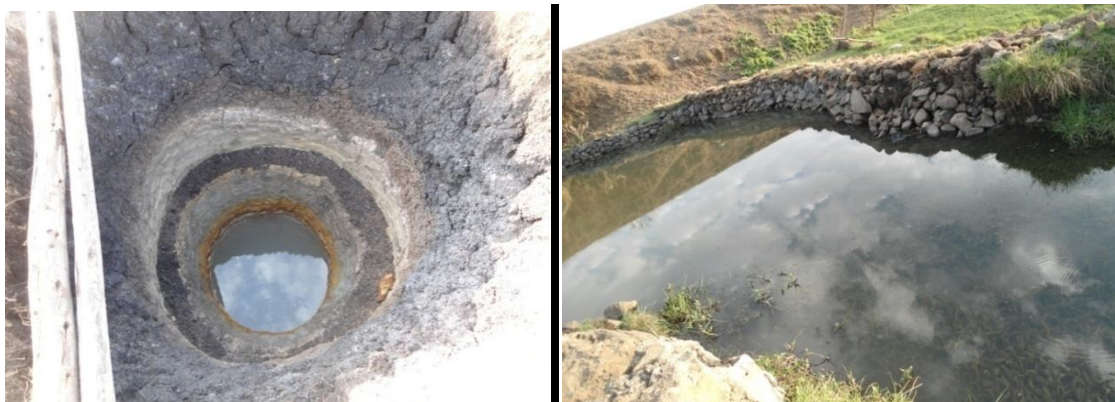
Fig5.9:-Hand-dug well constructed in SHH area to get the excess water (Field survey, 2014)
