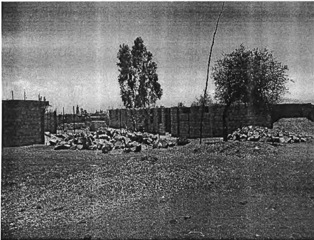
Fig.4. 2. Tede Dildima Kebele Health Center, under construction
