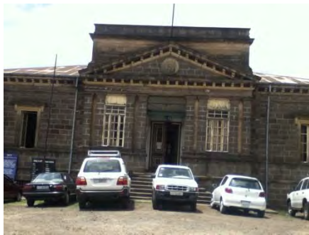
Bank of Abyssinia (Arda Sub-City)
