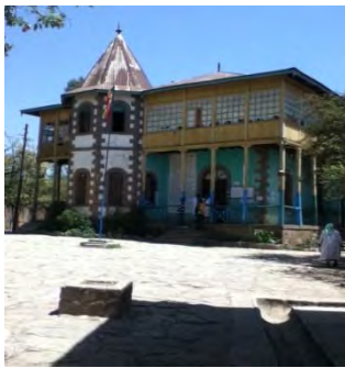
The front of the Building
