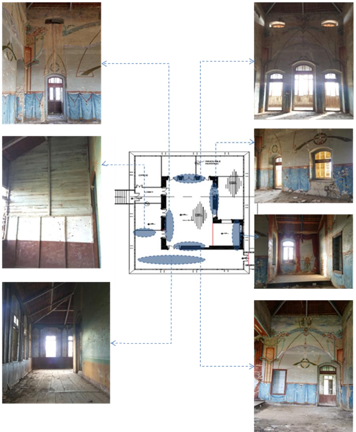
Figure 4.24 –interior wall condition first floor of Block A
