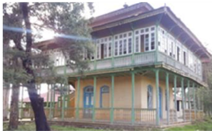
Wooden post and balustrades at block B
