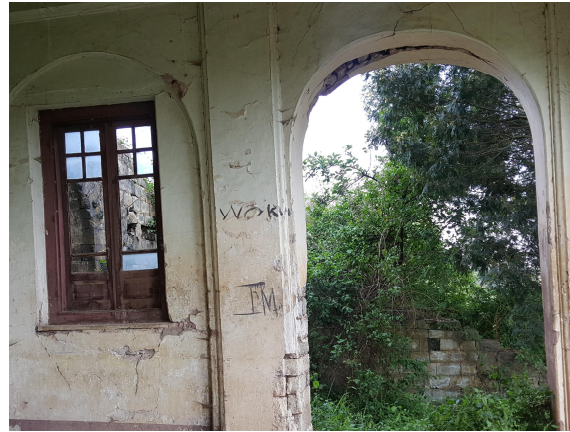
Figure 4.15 – masonry stair case to Block A upper floor, view from the corridor of block A at South West side.
