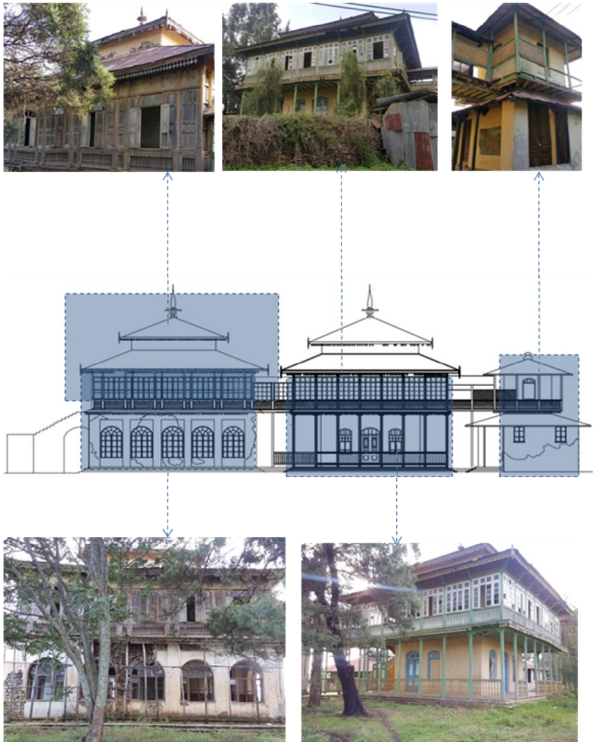
Figure 4.30 –exterior wall condition on north east elevation
