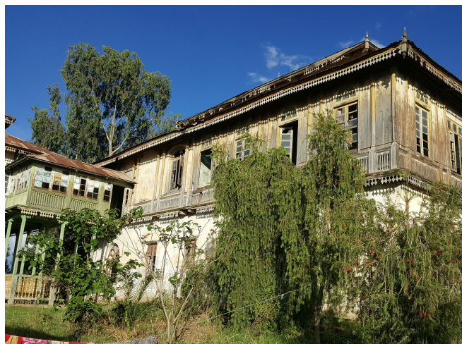
Figure 4.16 – timber framed glass wall of the upper floor of block A and connecting bridge to block B
