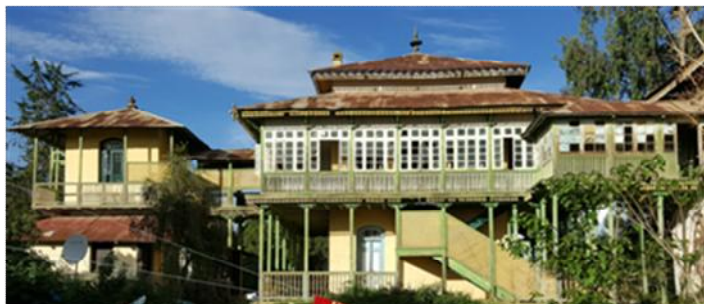
Masonry wall Wooden post and balustrades at block B and C
