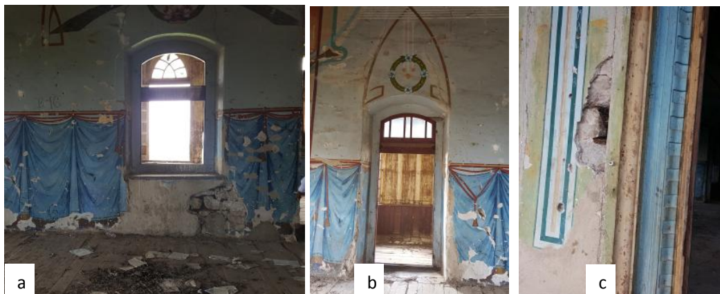
Figure 5.3 – hammering of nails on the wall surface
