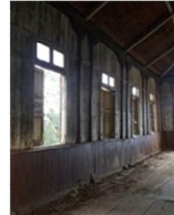
Wooden post as roof support at block A
