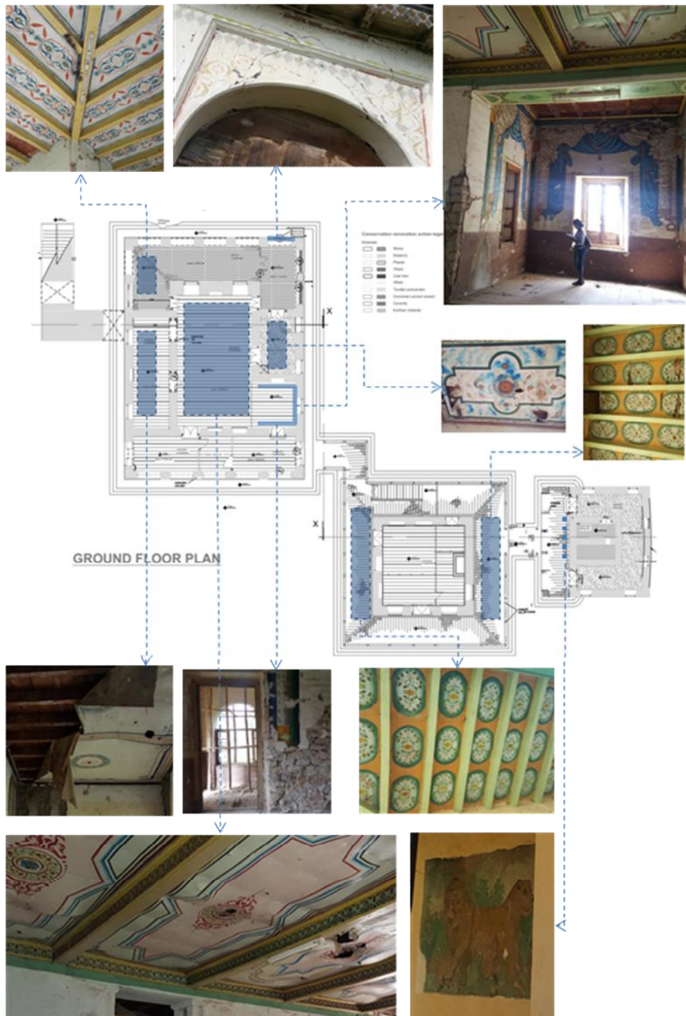
Figure 4.42 – wall and ceiling paint
