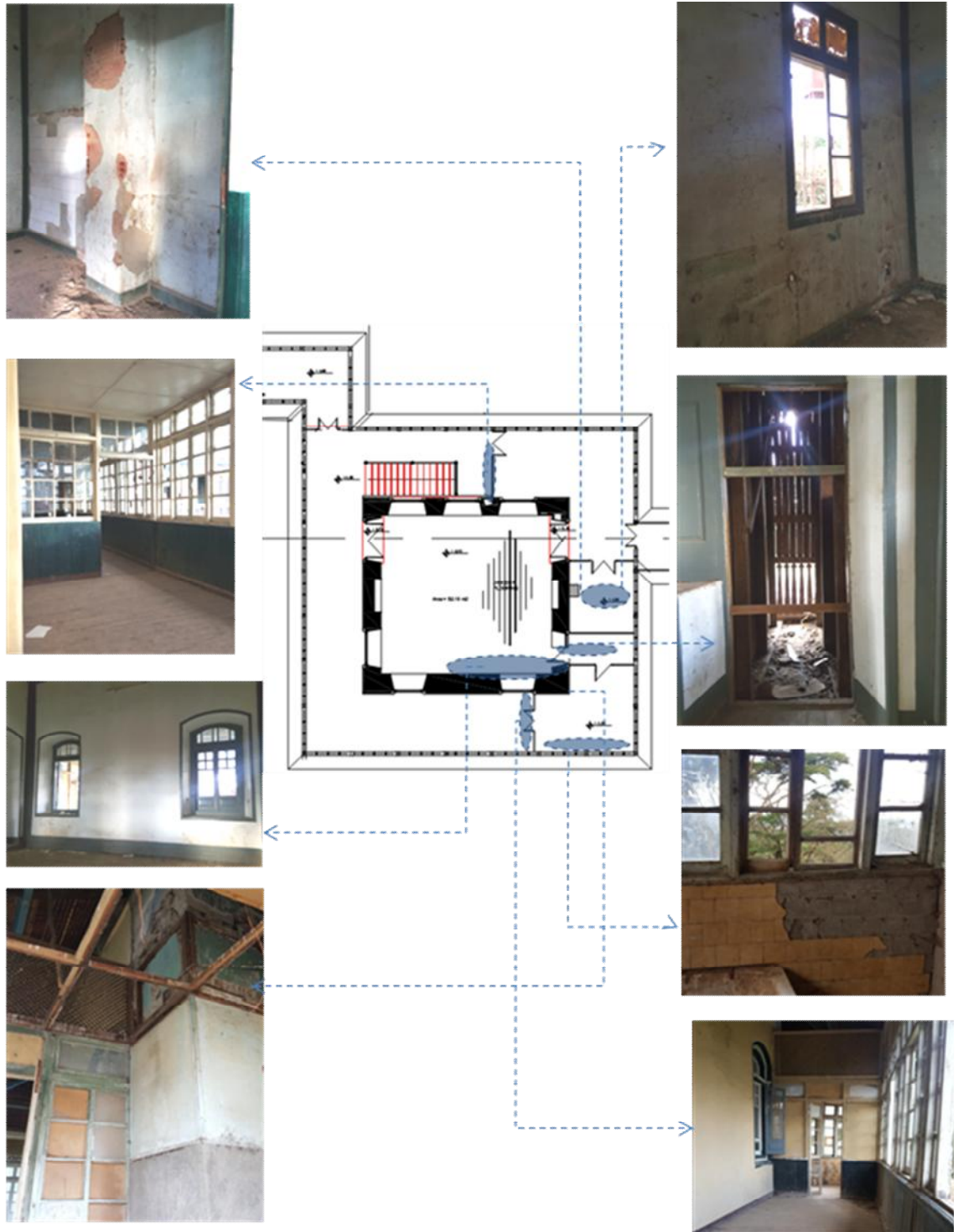
Figure 4.25 –interior wall condition first floor of Block B
