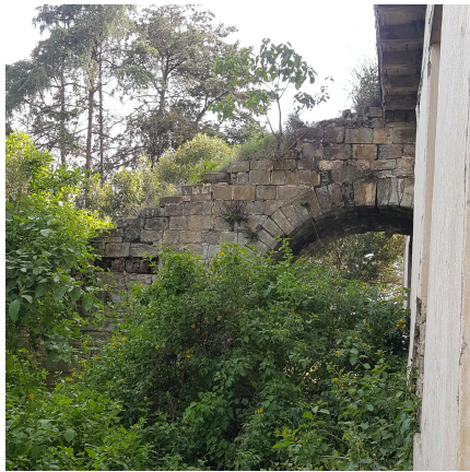
Figure 4.14 – masonry stair case to Block A upper floor , view from North East side of the Palace
