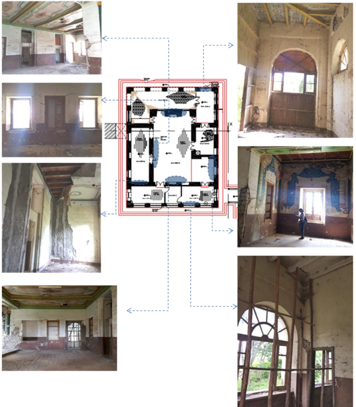
Figure 4.23 – Block A, ground floor interior wall condition
