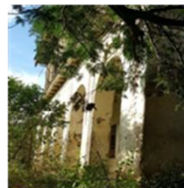
Column at block A
