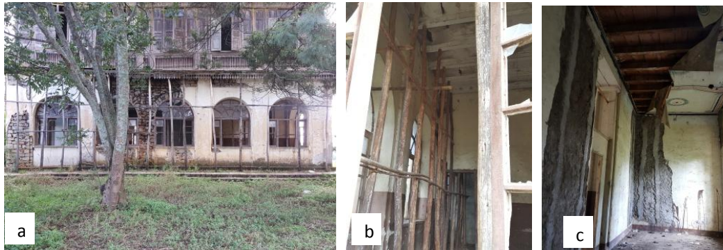
Figure 5.2 – consolidation intervention on the building
