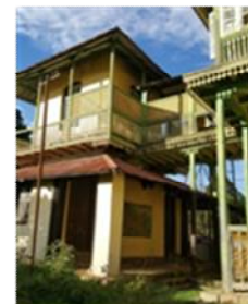
Column and Wooden post at block C
