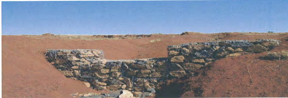
Figure 9: Gully rehabilitation by stone check dam (own photo at the field)
