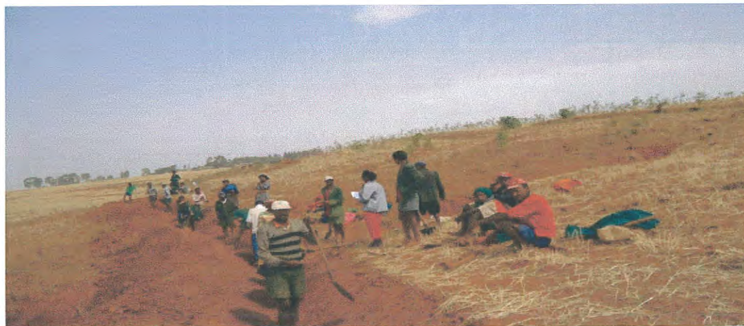
Figure 10: Construction of cut off drain during field observation (own photo at the field)
