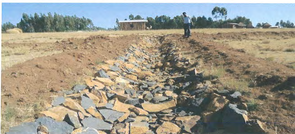
Figure 11: Well constructed stone paved waterway (own photo at the field)
