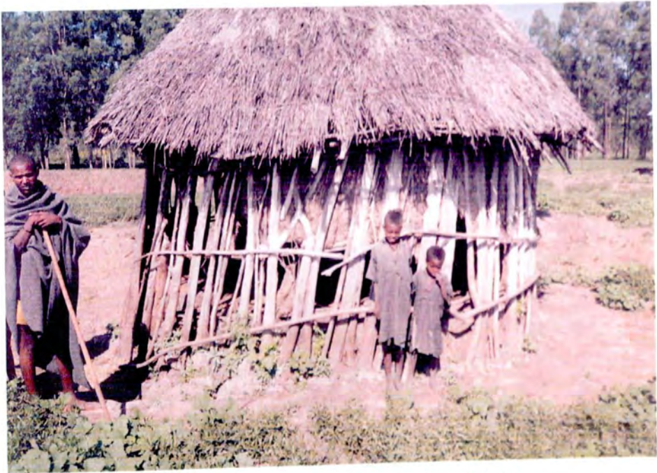
Photo 5.2 Damaged hut in Shina TSION kebele
