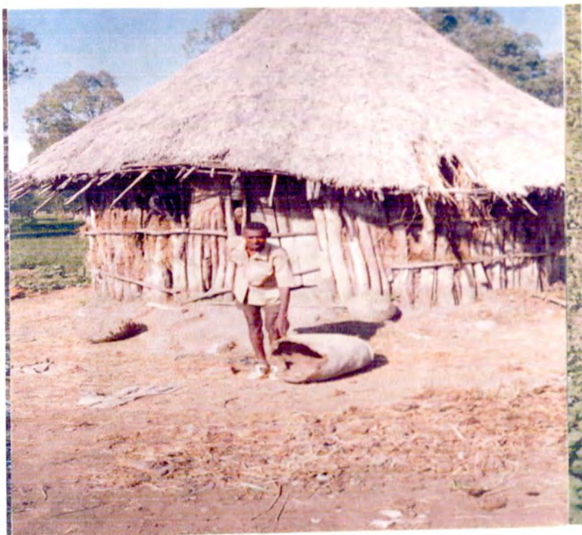
Photo 5.3 mud plaster grain container damaged by floodwater
