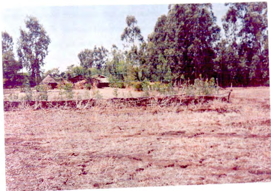
Photo 5.6 Earthen levee in Deber Zuria Adisge kebele
