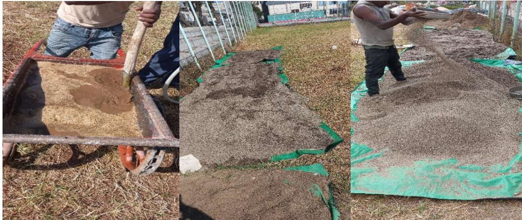
Washing, drying and sieving of fine aggregate
