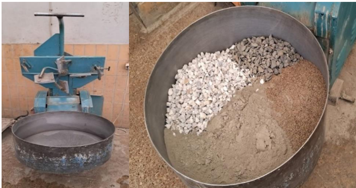
Figure 3.10 Drum mixer along with materials ready for mix
