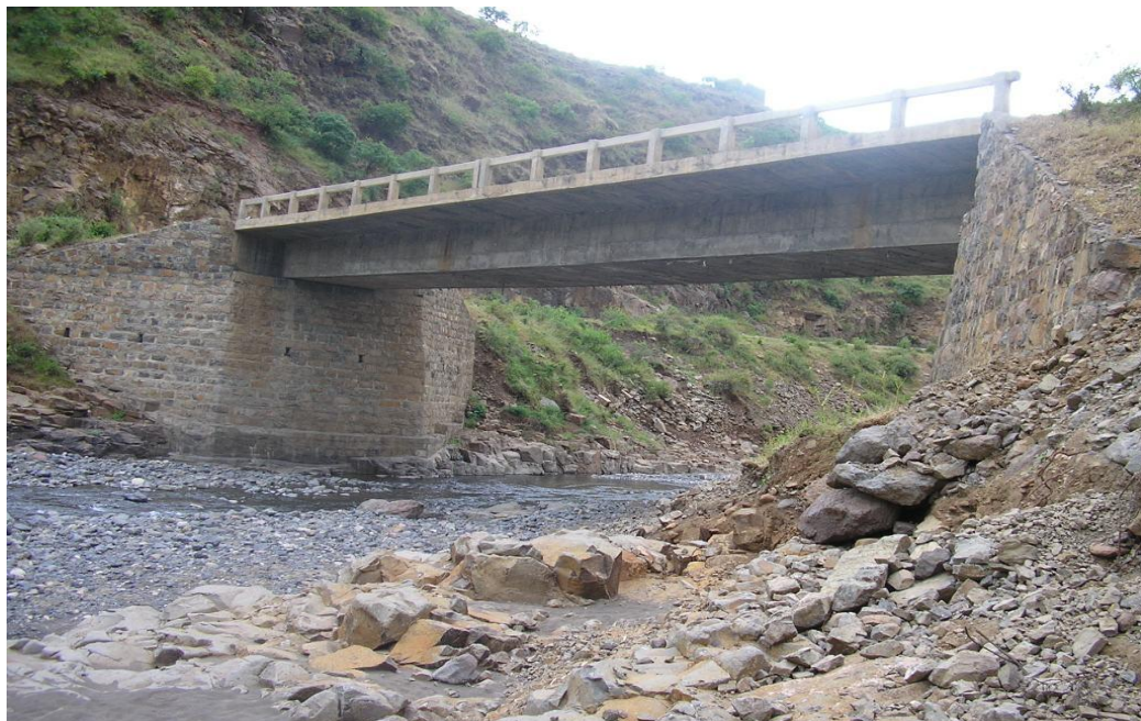
Figure 3.2 Koga River Bridge
