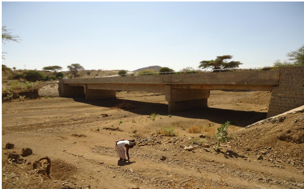
Figure 3.9 Meterie River Bridge
