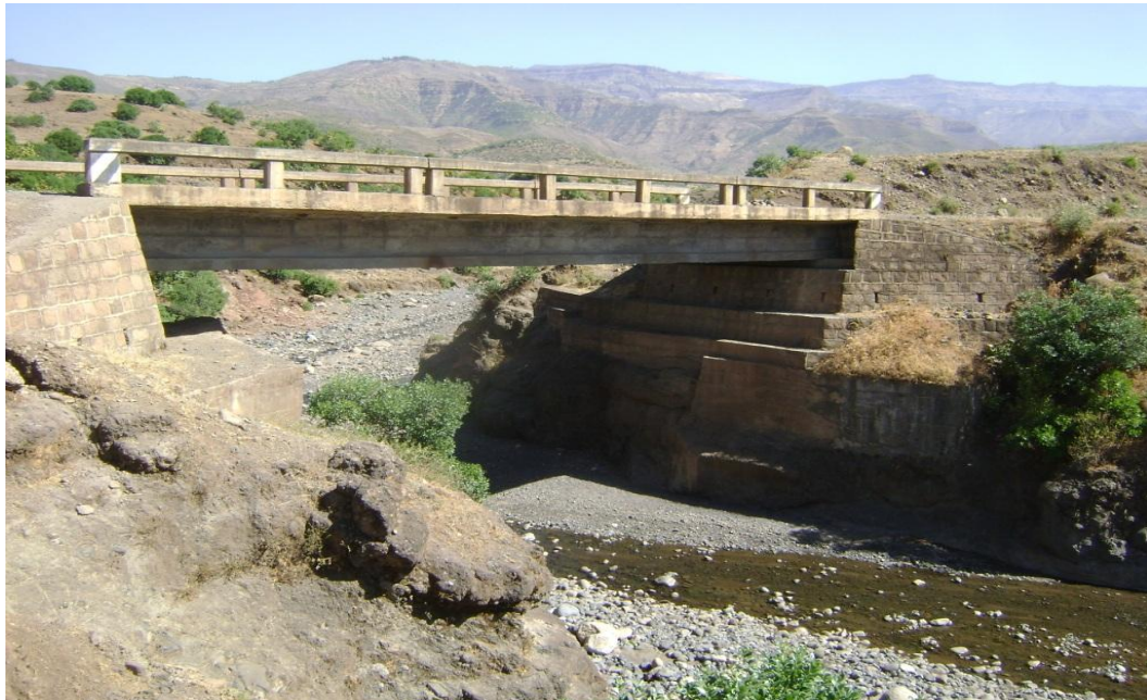
Figure 3.8 Semeno River Bridge
