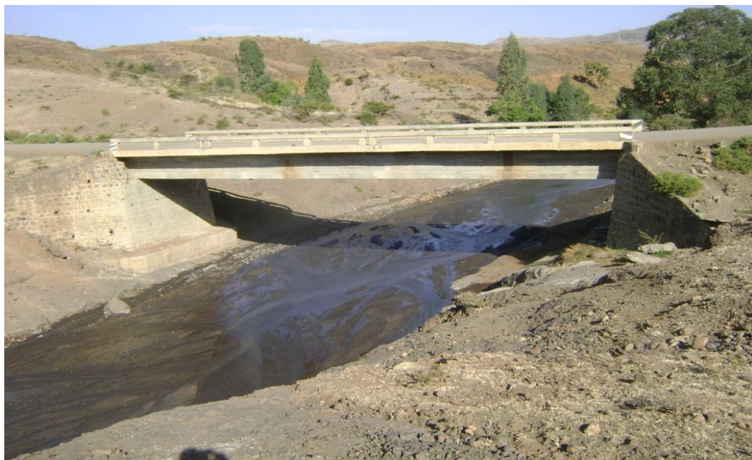
Figure 3.6 Warkena River Bridge
