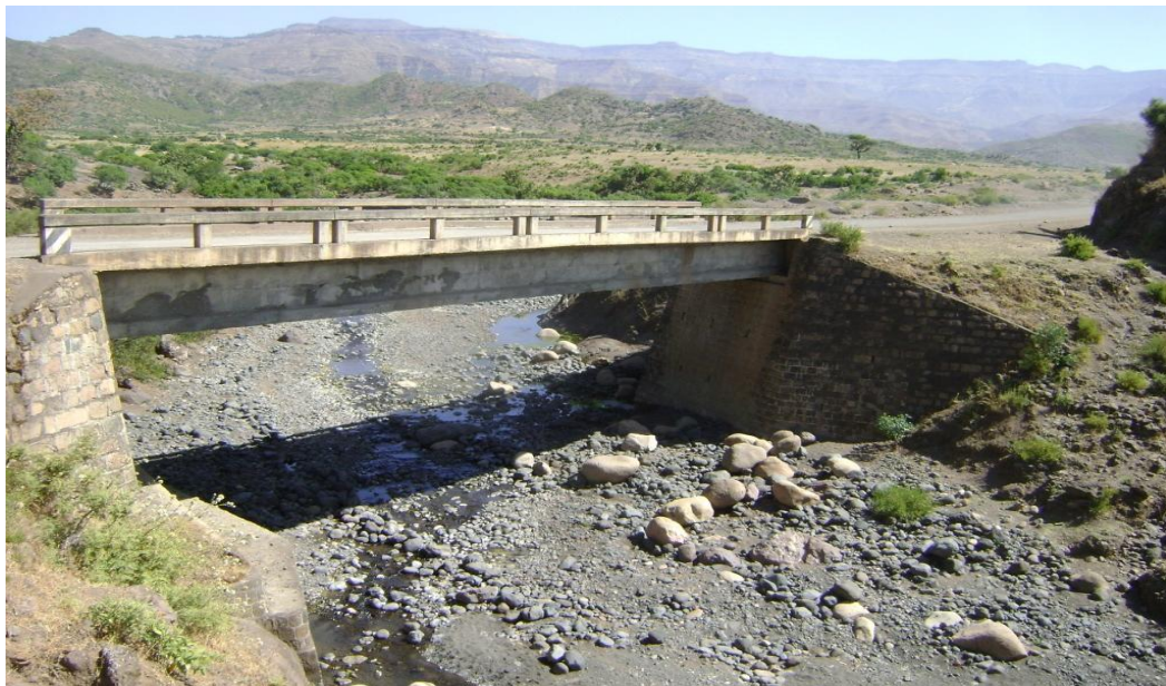
Figure 3.1 Abiya River Bridge
