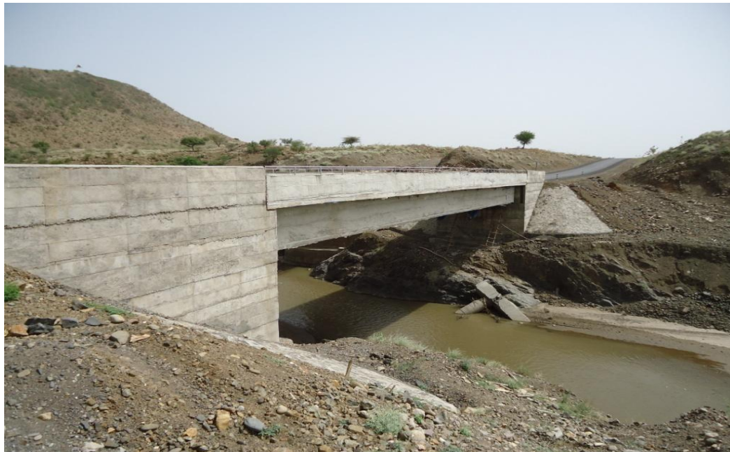
Figure 3.5 Burure River Bridge
