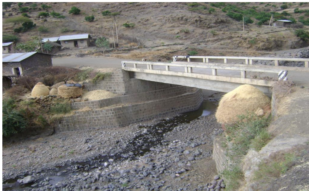
Figure 3.3 Dilbazia River Bridge
