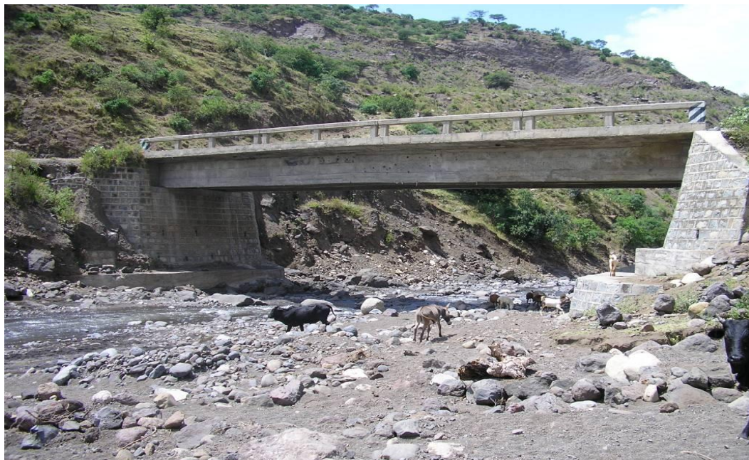
Figure 3.4 Teda River Bridge
