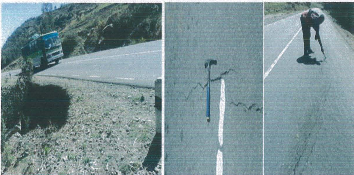
Figure 1.1 Slides showing views of landslide effects at the main asphalt road of the site.
