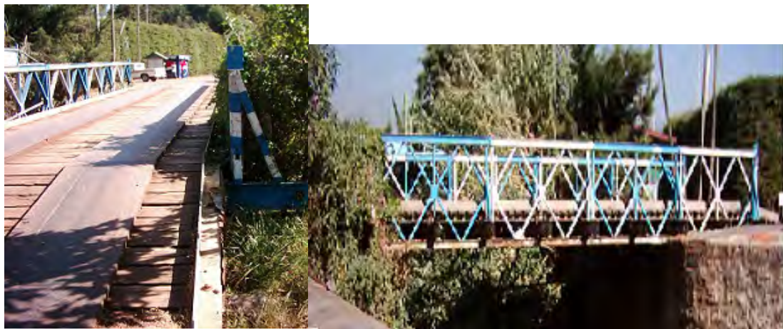
Figure 4.1 Baily bridge at the entrance to the Addis Ababa Tennis Club
