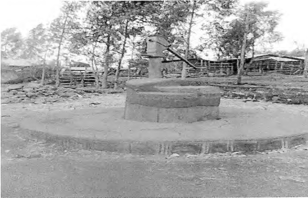
Figure 5: Non-functional scheme, Problem of depth and with out fence for HDW, Dugmasefer Gote , Berber kebele
