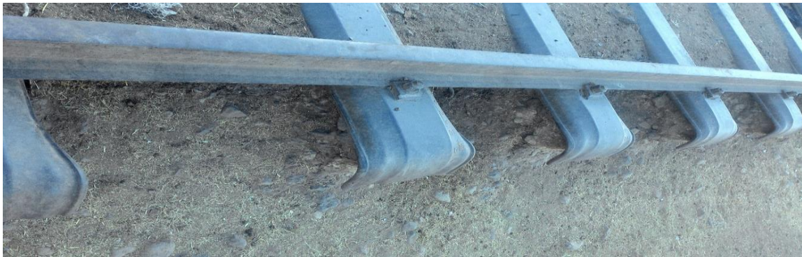
Fig. 3.6. Fouling condition of old rail track ballast Lagahar-Akaki section
