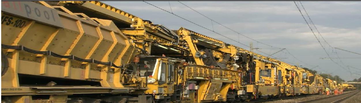
Fig. 4.2 Self-propelled ballast recycling machine
