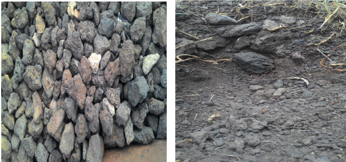
Fig.3.3. Unfouled and fouled ballast of old Ethiopian railway
