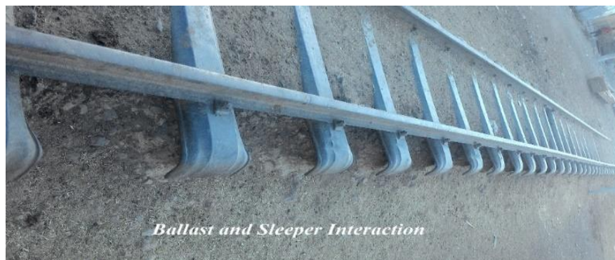
Fig. 3.5. Ballast and sleeper contact lose condition at Lagahar-Akaki section
