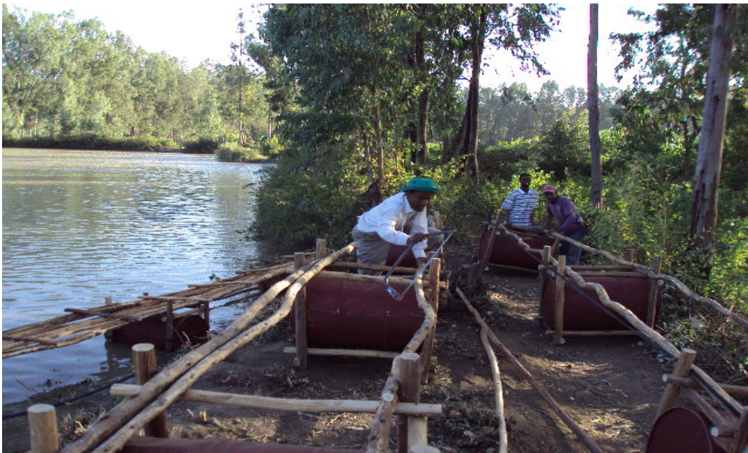
Plate 2. Landing stage construction (December, 2010)
