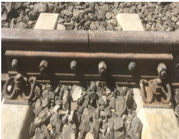
Figure 4.1: Fish plates, bolts, nuts and rail clips
