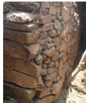
Un-mortared dry masonry wall built at Arhata
