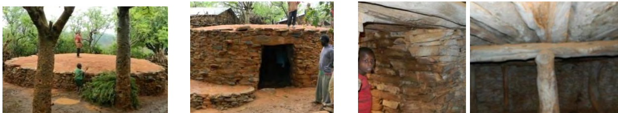
The rammed roof top, Main entrance and exit of Kimbilita Paffta The interior pictorial presentation of Kimbilita paffta
