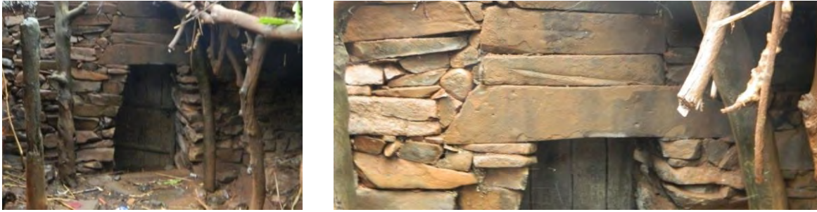
Picture 5.24 Pictorial analysis of entrance and exit ( Harra ) of the kimbilita Kossa and it telling us the main entrance of Kimbilita Kossa , un mortared dray masonry wall surface and shown supporting stone lintel; the rammed clay roof surface which is used building Manna and Kossa supported by wooden beams and columns. Kimbilita Kossa built in the lower sloppy ground level of Tikka .
