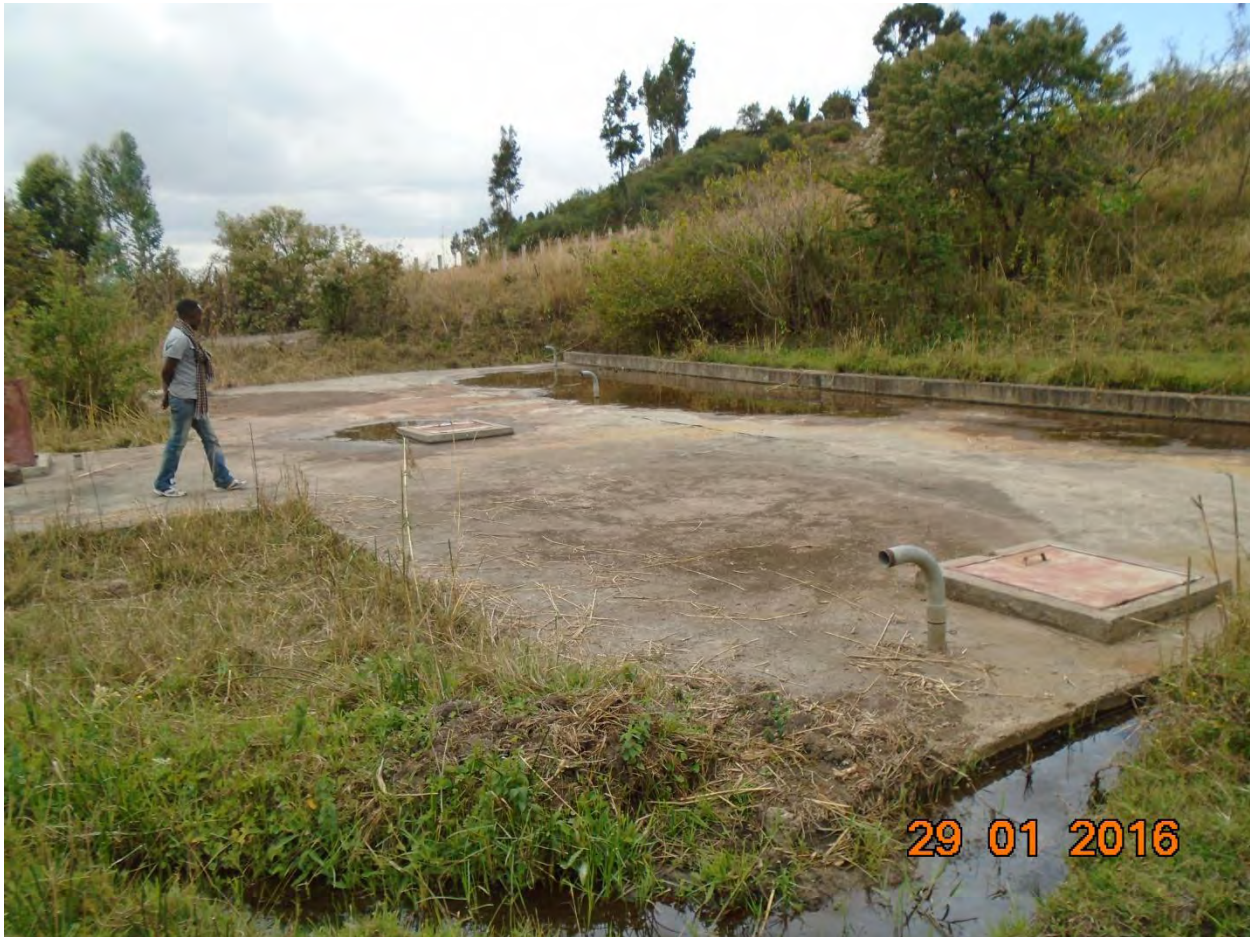
Figure 3: Makecho Spring capping structure.
