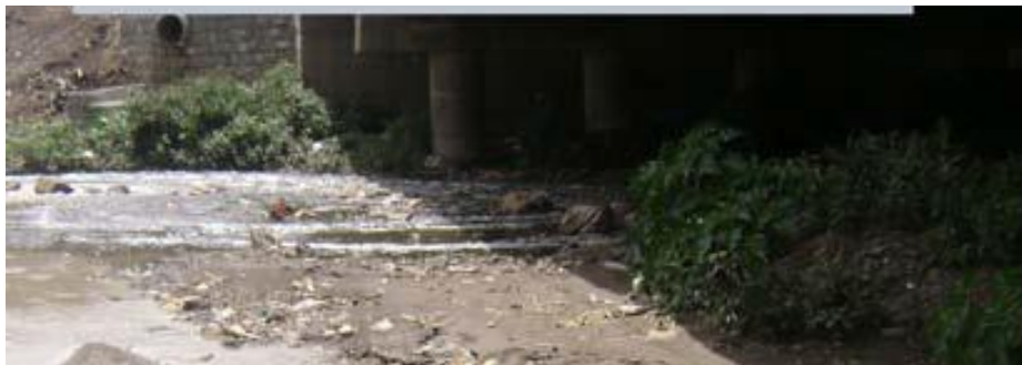
Figure 4.6: Little Akaki river drainage
