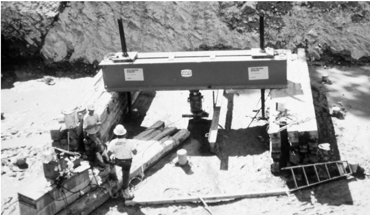
FIGURE 12.19 Micropile load test. (From Hayward Baker Inc. With permission.)
