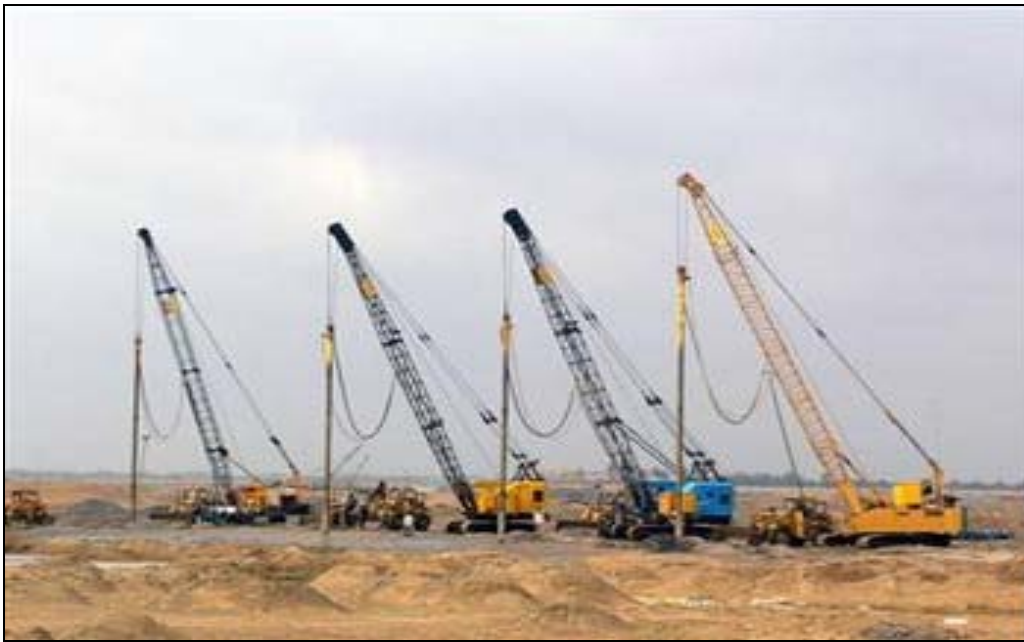
Figure 7. Installation works for the tank farm at Paradeep, India
