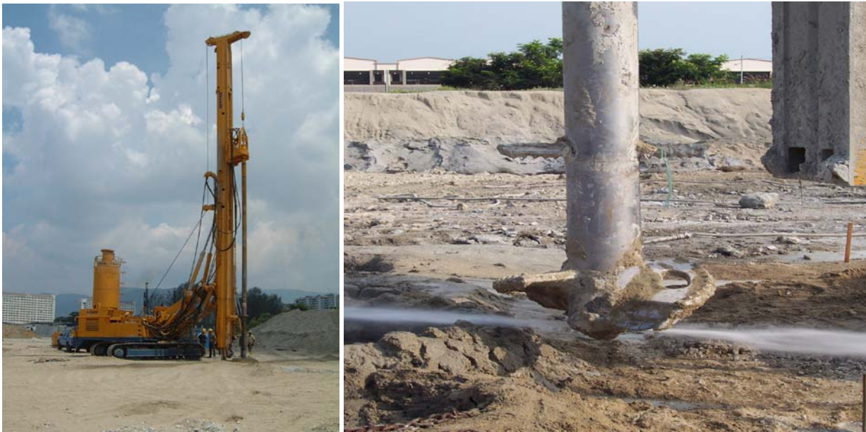
Figure 3.2: Deep soil Mixing works at Jelutong Sewage Treatment Plant
