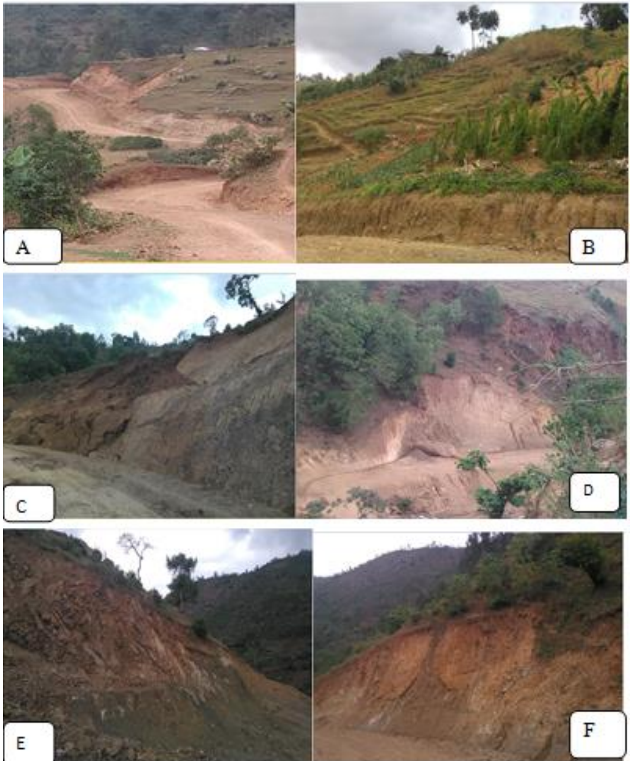
Steep slope cut (A, C, D and F). Cultivation on slope face (B). Quarry (E).
