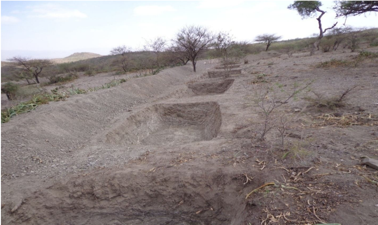
Figure 5.3 Structural conservation measures on the side of mountain
