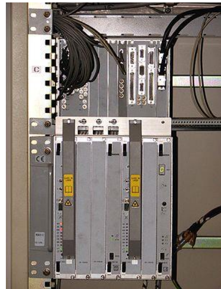
Figure 2.6: Add-Drop Multiplexer [15]
