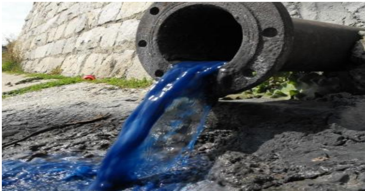
Fig3. Textile wastewater discharged to the environment without treatment (Tripathy, 2013)
