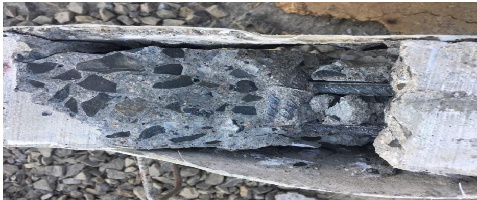
Figure 4-13 De-bonding of GFRP and crushing of concrete
