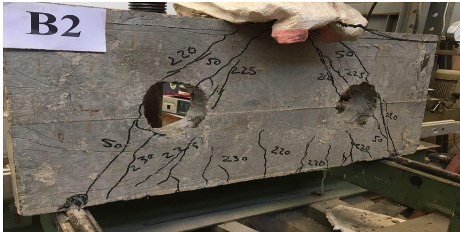
Figure 4-10 Flexural and shear cracks of B2
