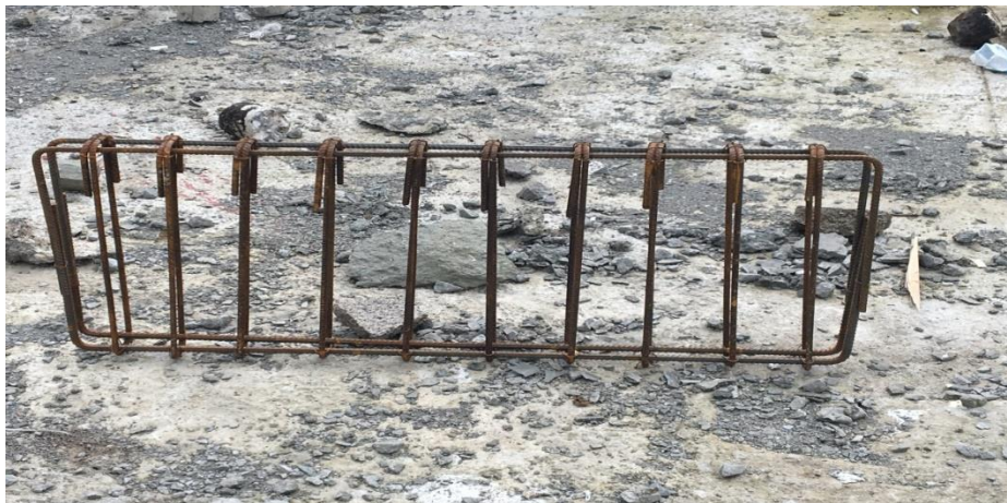
Figure 4-2 Fixing for tension, compression and shear reinforcements
