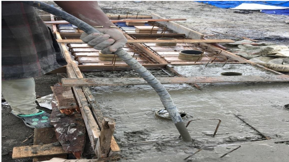
Figure 4-1 Compaction of concrete with a needle vibrator
