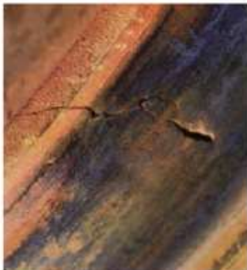
Figure 10: Fatigue crack on the tread propagated from thermal crack [43]
