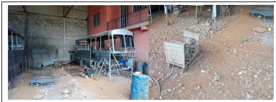
Figure 4.3welding process and machine (Field survey)
