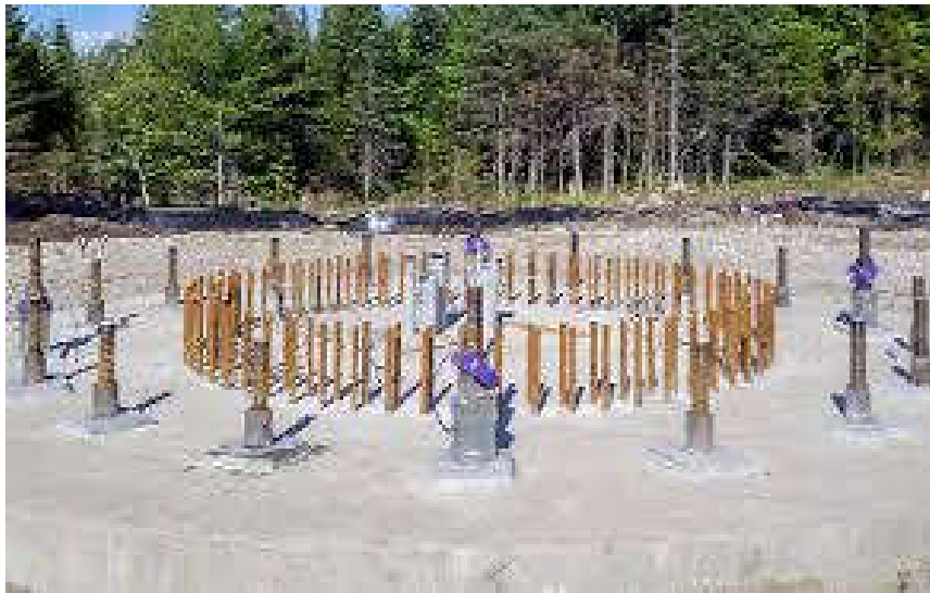
Figure 6: Rock anchor foundation (Miceli, 2012)
