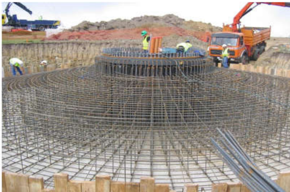
Figure 5: Anchor cage foundation (Miceli, 2012)
