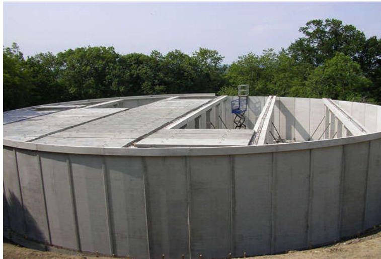
Figure 7: Precast concrete foundation (Meceli, 2013)
