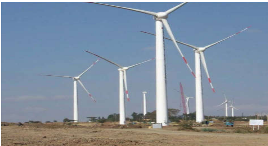
Figure 10: View of Some completed Wind Turbines (Adama I Wind farm Project Summary Report, 2010)
