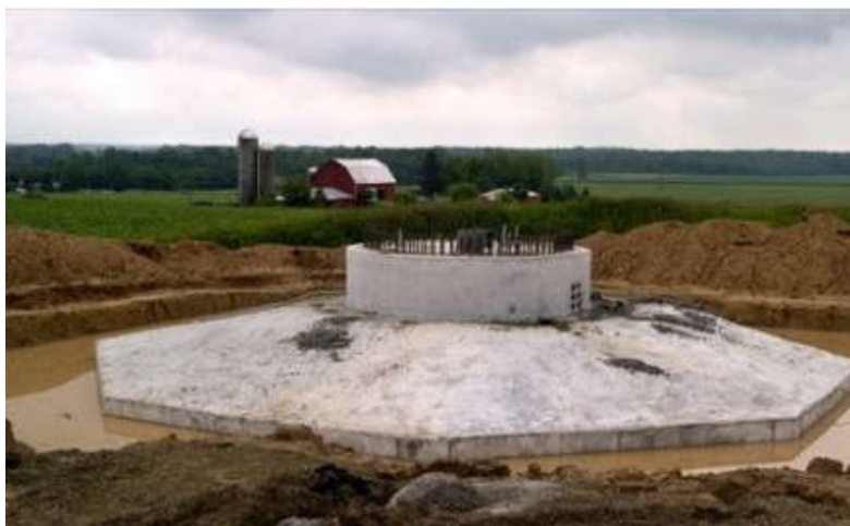
Figure 4: Octagonal gravity base foundation
