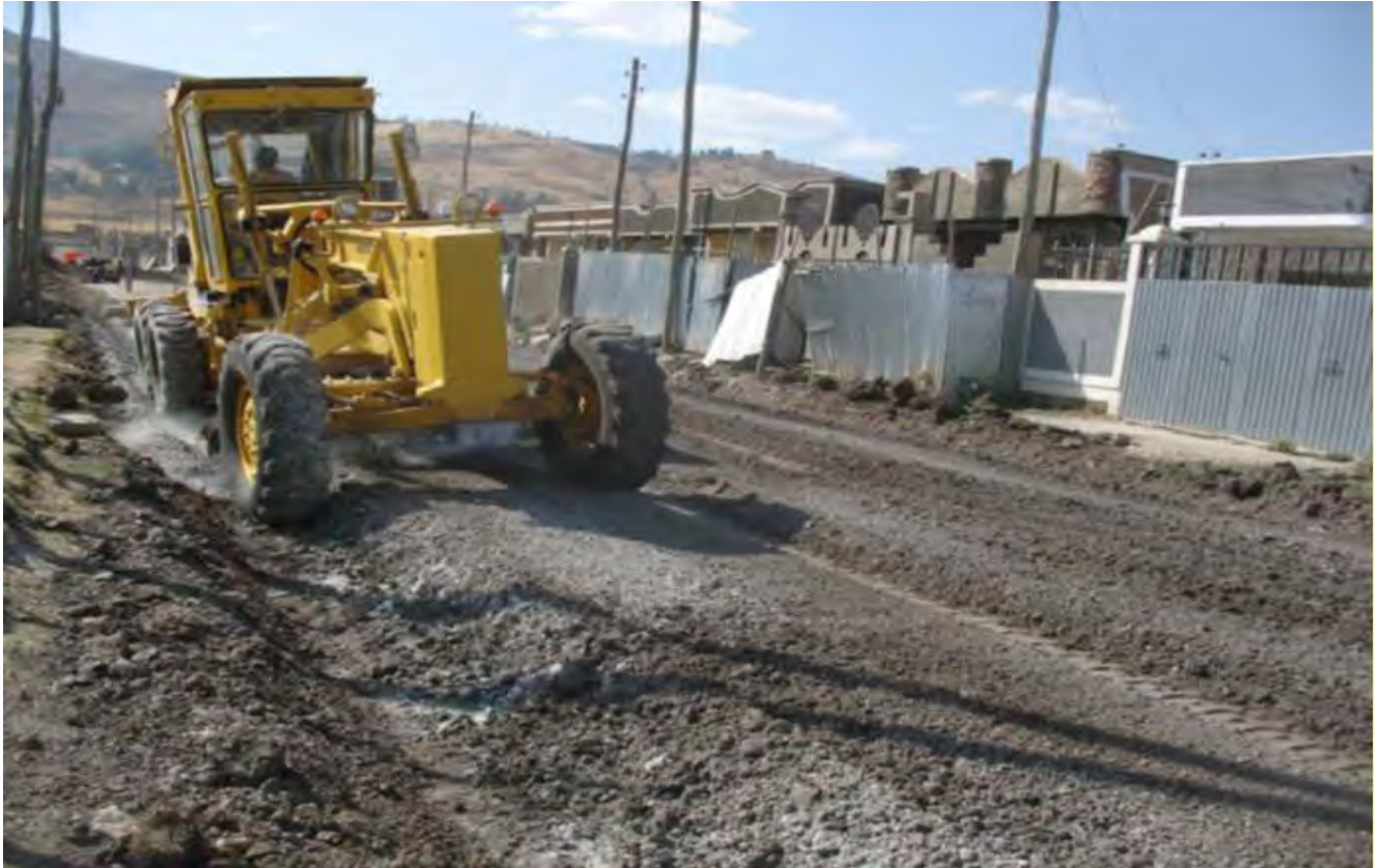
Figure 8: Creating Drainage
