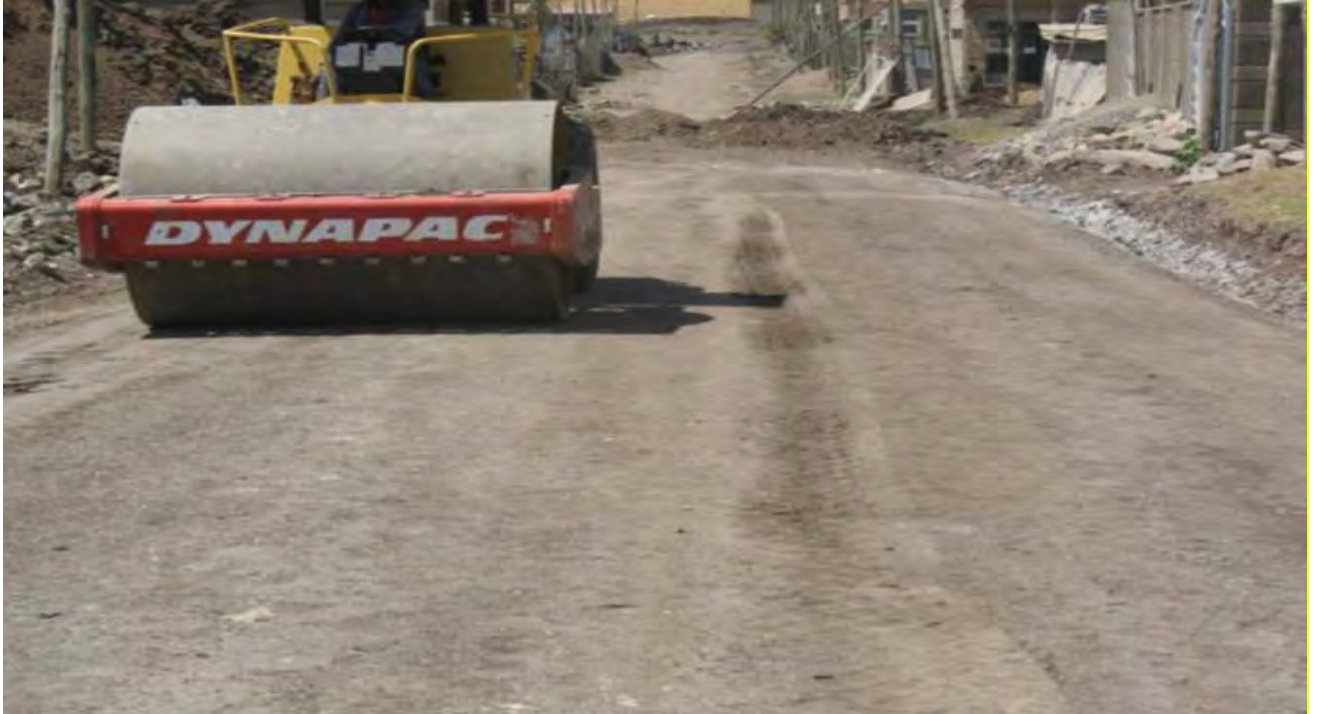
Figure 15: Compaction
