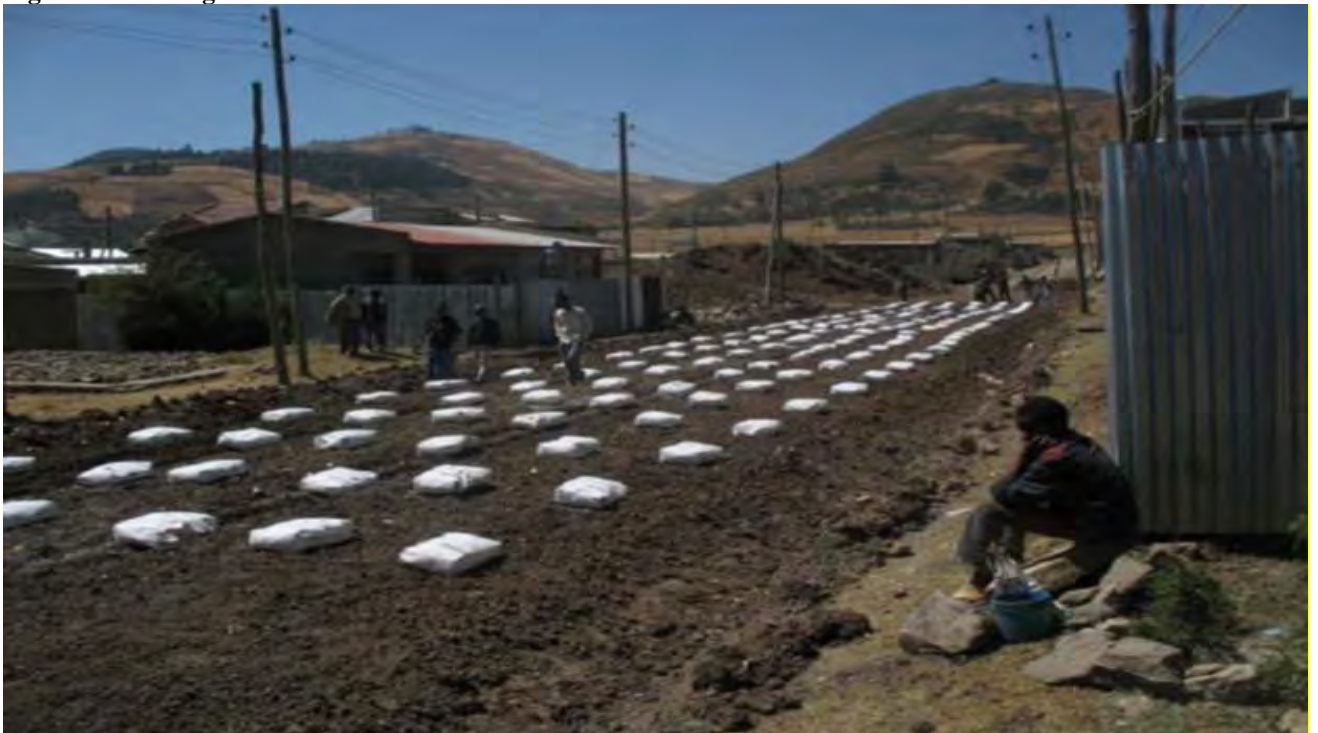
Figure 10: placing product as per the spacing (the markings)
