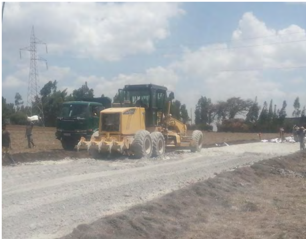
Figure 25: Mixing on site
