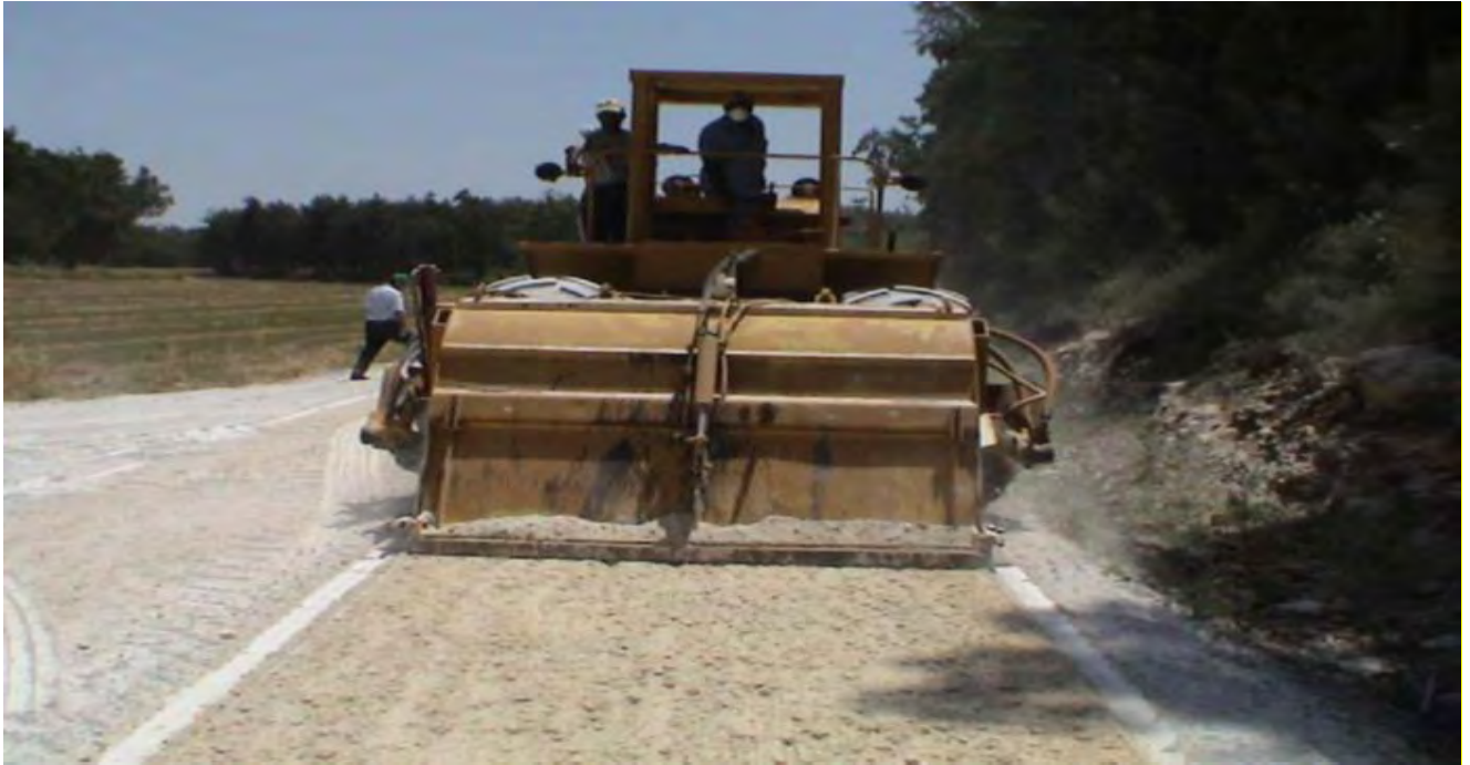
Figure 12: Dry Mixing
