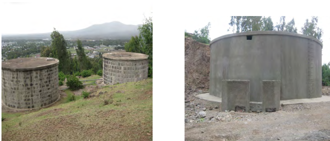
Figure 5: Old and newly constructed municipal water reservoirs, Dukam, 2010.
