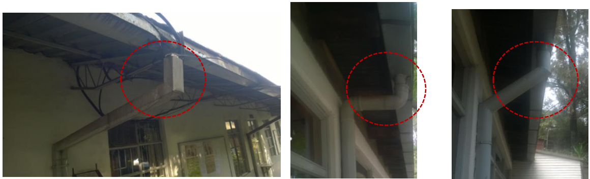
Figure 25: Types of bended rectangular and circular downpipe on EiABC buildings
