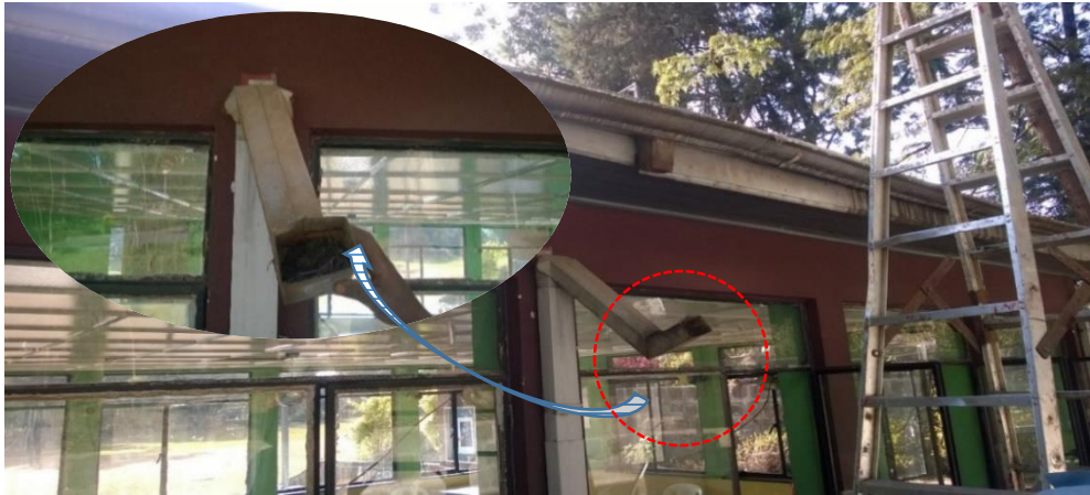
Figure 28: Dismantled downpipe system on student cafe
