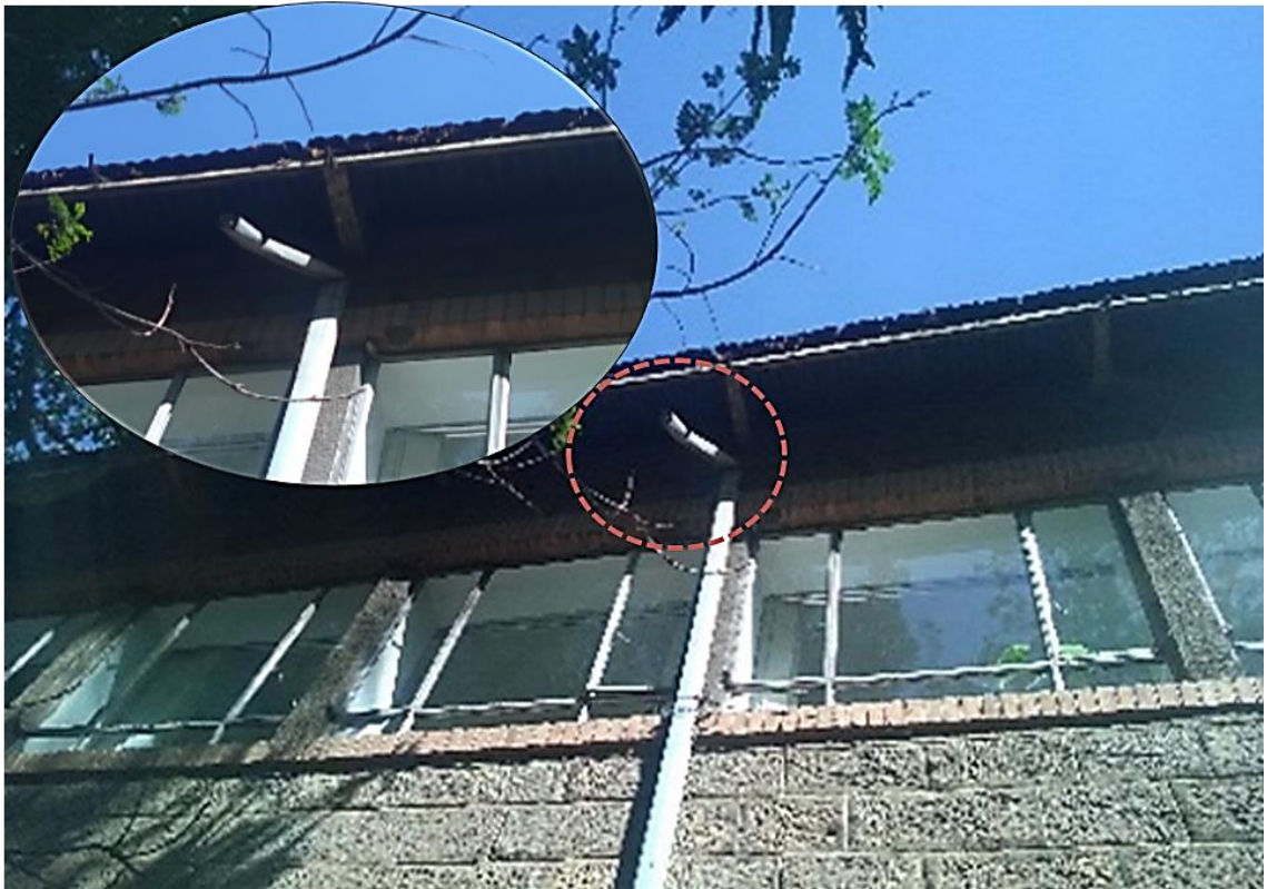
Figure 14: Trapezoidal gutter system on administration building
