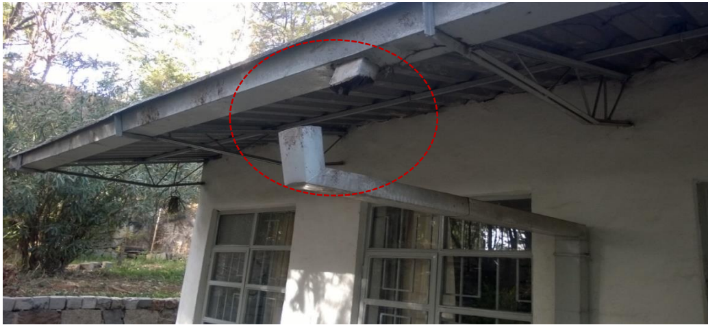
Figure 26: Dismantled downpipe on finance buildings
