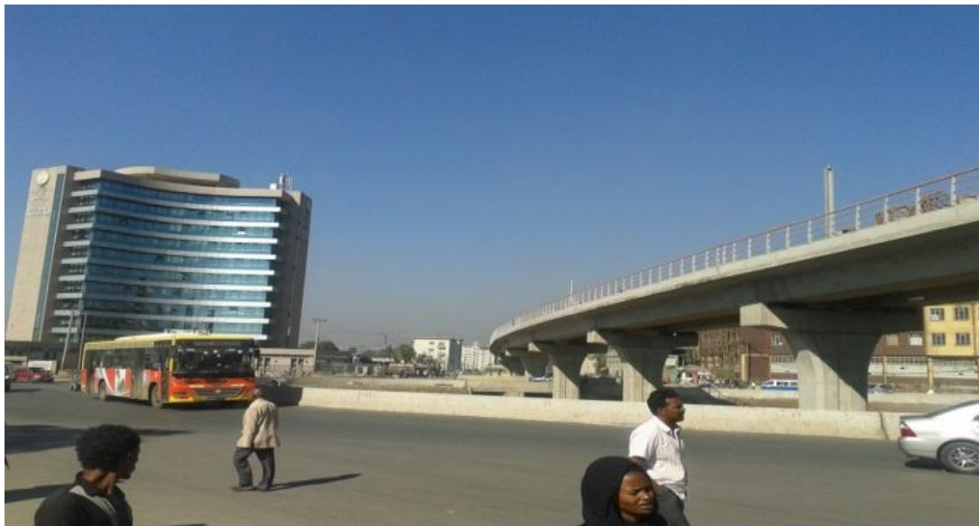
Figure 1.2: on progress AALRT rail project Mexico area.
