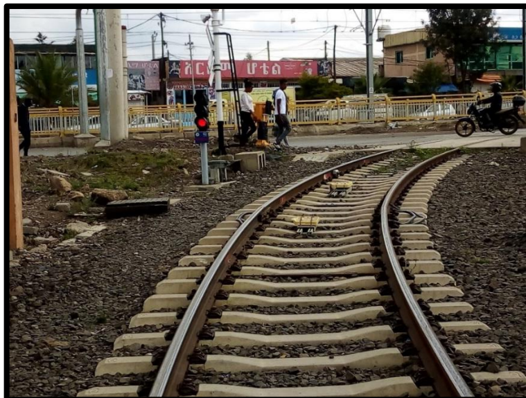
Figure 4. 8: Level crossing at AALRT Kality
