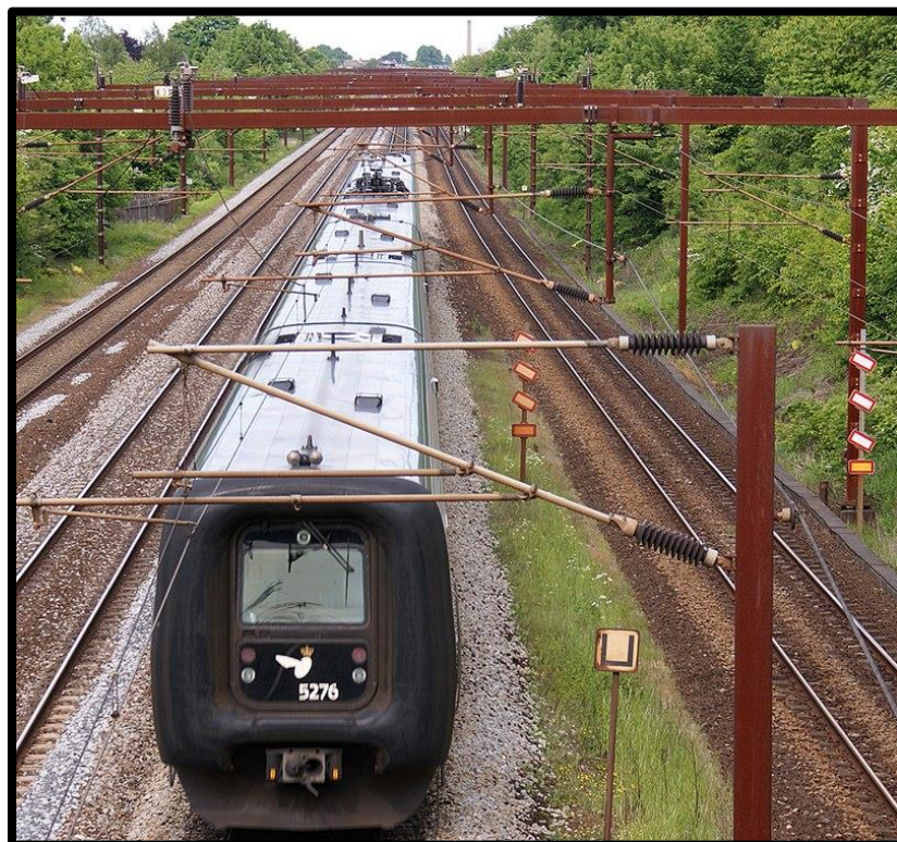
Figure 1. 3: Showing movement of overhead line on train [8]
