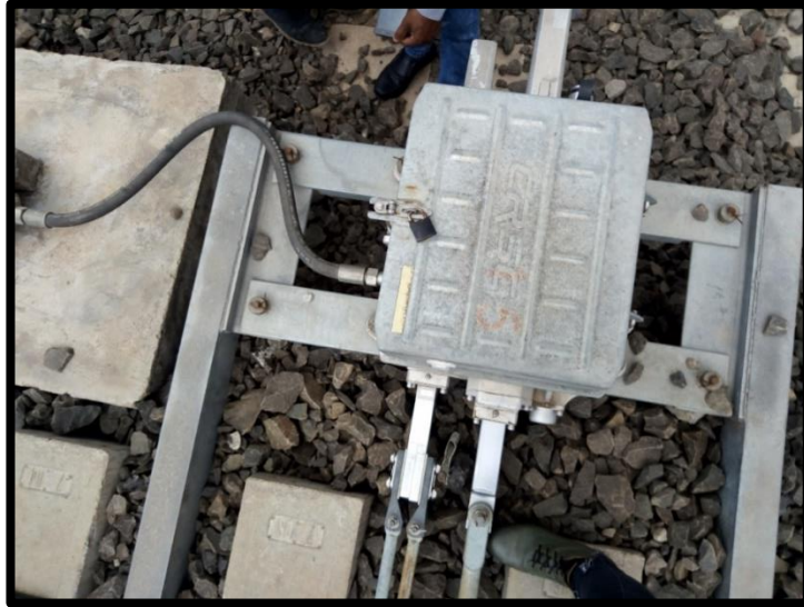
Figure 4. 9: Point machine top view
