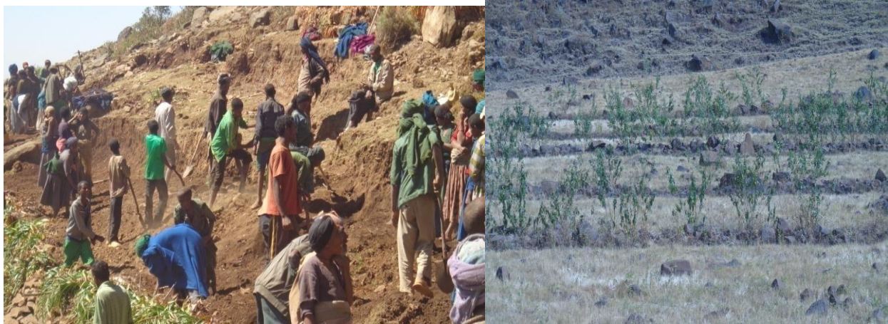
Figure 3.8: People constructing terraces in Chefakit kebele (left) and a rare case of successful model terraces with planted trees along the terrace in Butila kebele (right)
