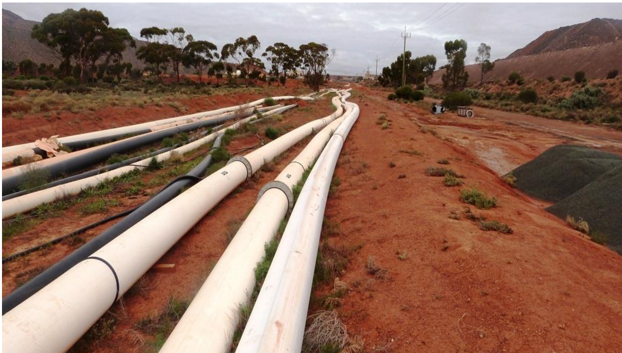
Image 2:- Ethiopia-Djibouti natural gas pipeline under construction
