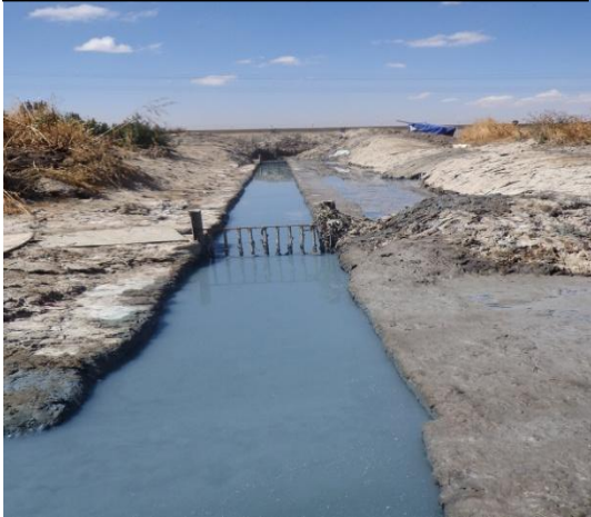
Openly left screenings near screens
