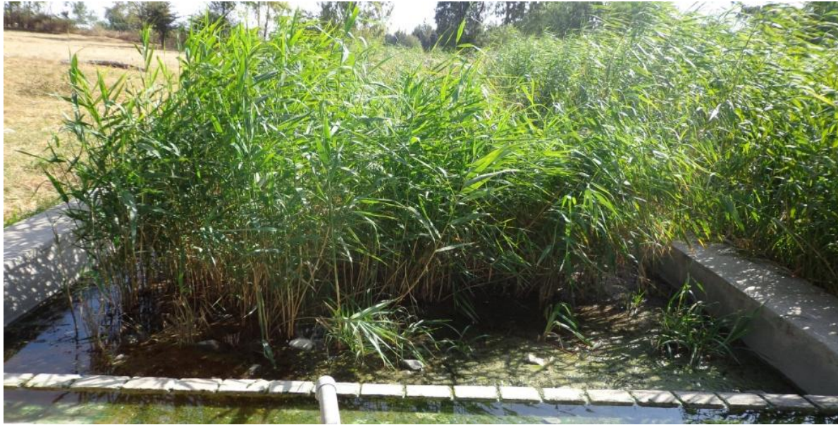
Figure 2.8. Free water surface type constructed wetland being used for tannery effluent treatment in Modjo Tannery, Ethiopia (actual field visit photo)
