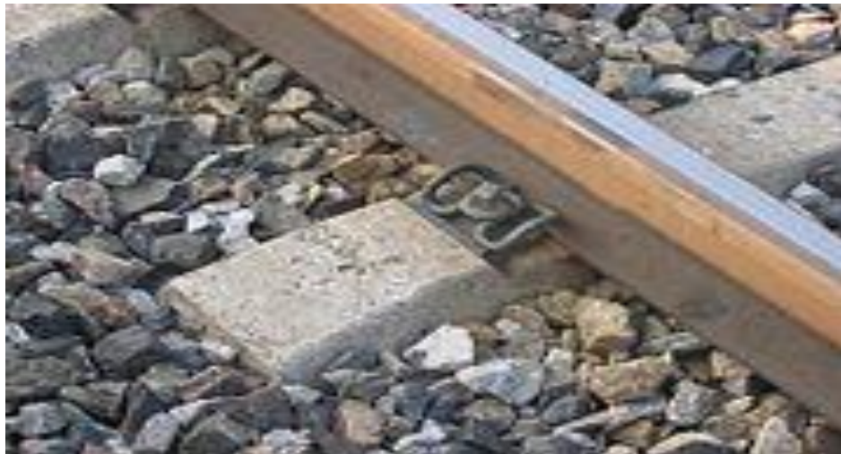
Figure1.6 Tension clamp fastening
