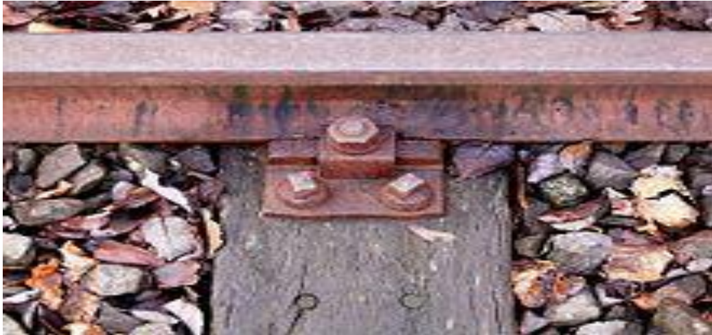
Figure 1.6 Rail to wooden sleeper fitting
