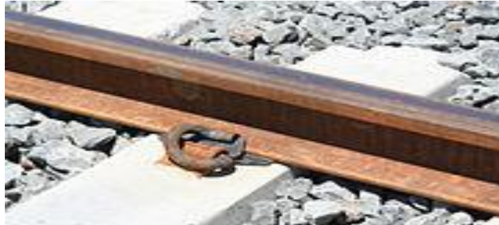
Figure 1.5 Pandrol's clip fastening
