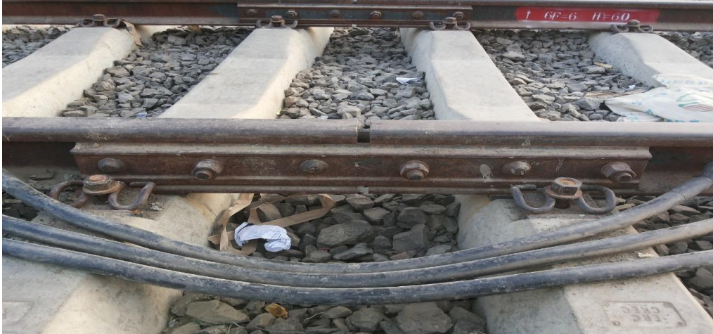
Figure 1.2 Standard rails fastening of Addis Ababa LRT.
