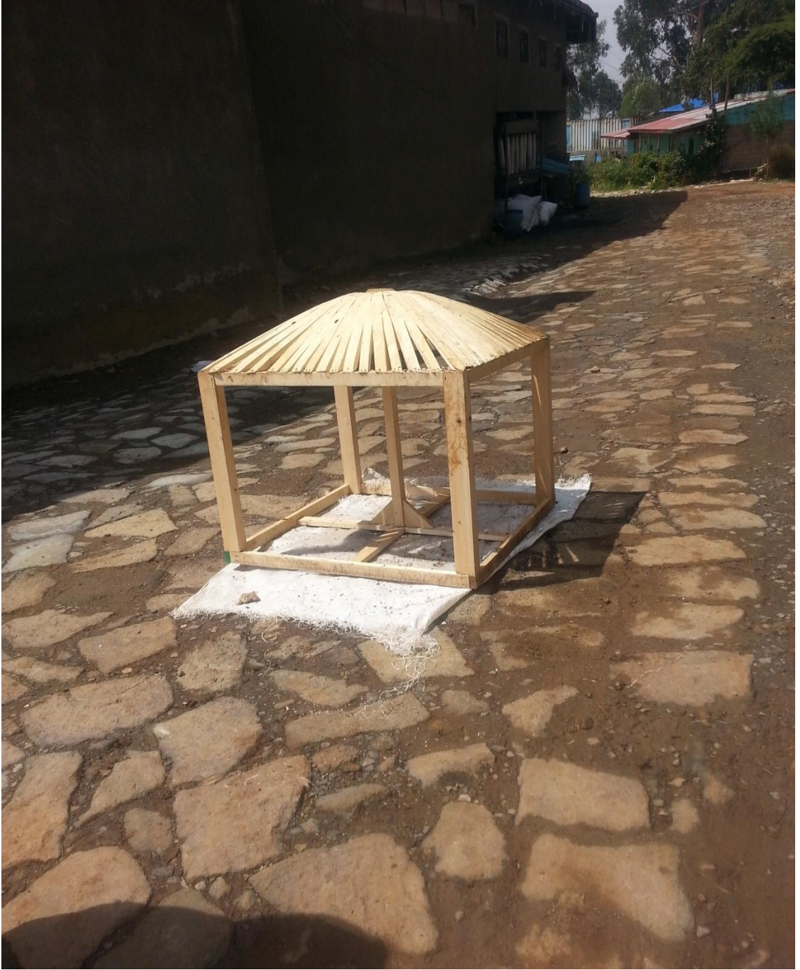
Figure 6. Dome type Dodeca Wooden Frame
