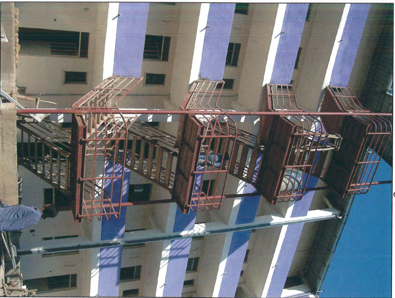
Stair case for G+4 Bldg.
