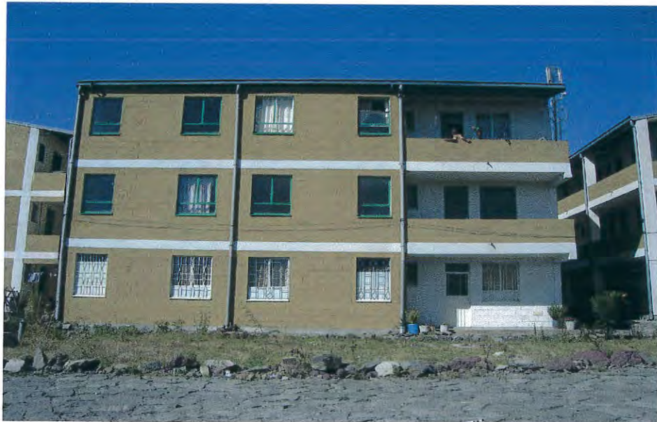
Photo of one of the GTZ 1 st phase condominium houses.
