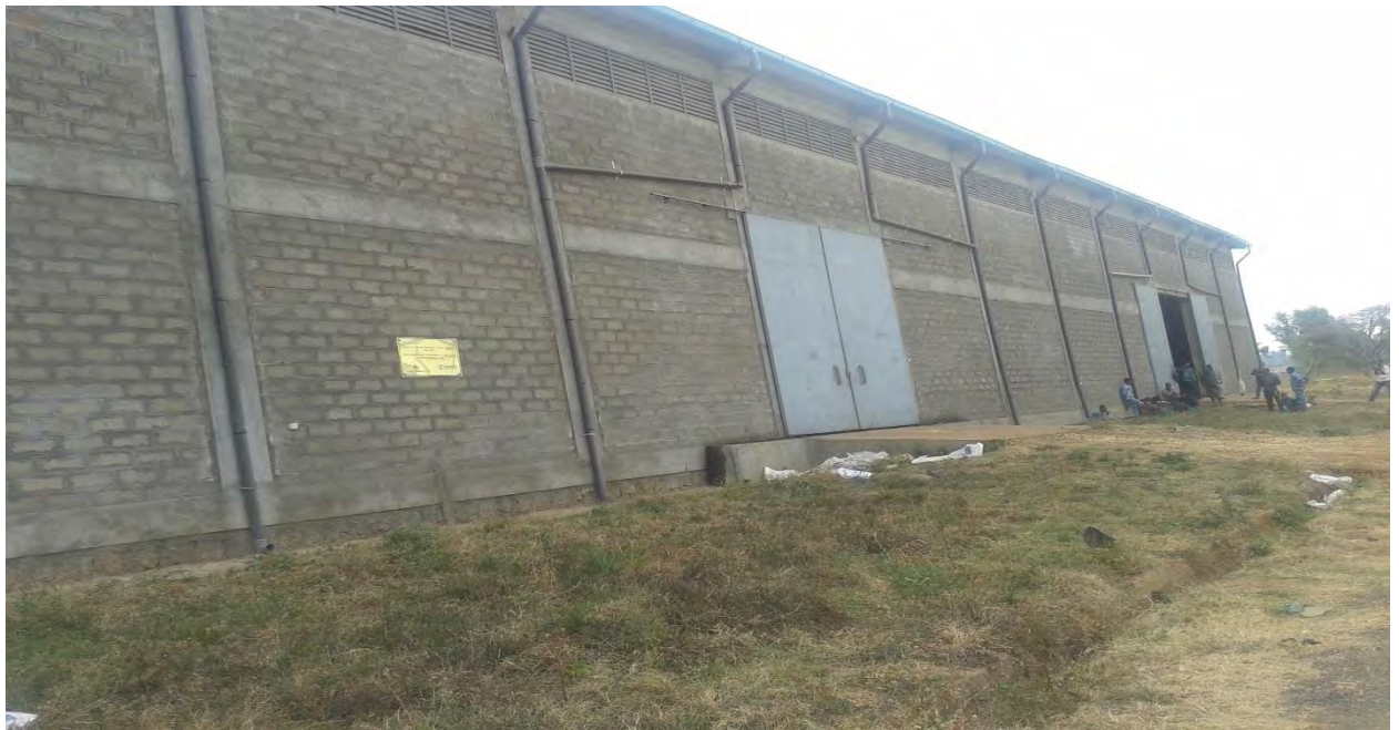
Photo 10. Gibe Dedessa grain warehouse
