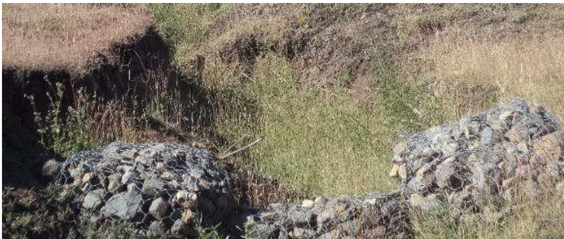
Figure 4: Stone check dam constructed to protect gully erosions
