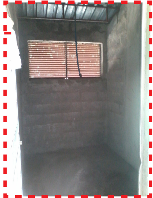
Fig. 6.8 Inside of a storage room of communal building in Gerji
