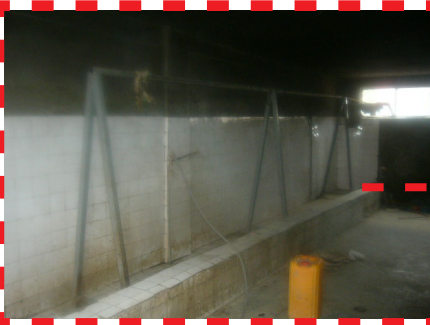
Fig. 8.29 Inside the slaughtering room
