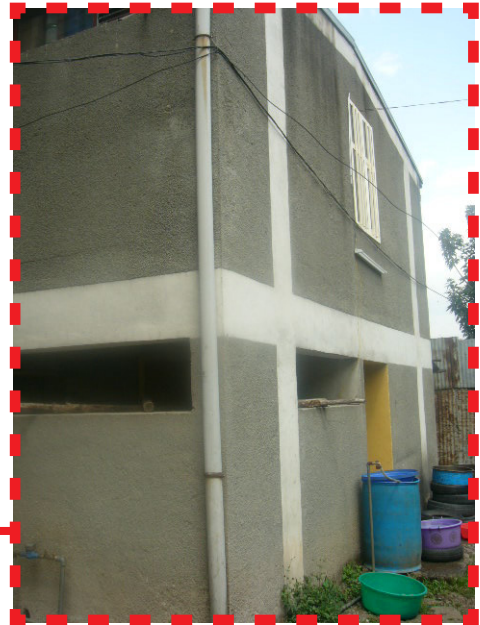
Communal building two located at a corner near Block 4.
