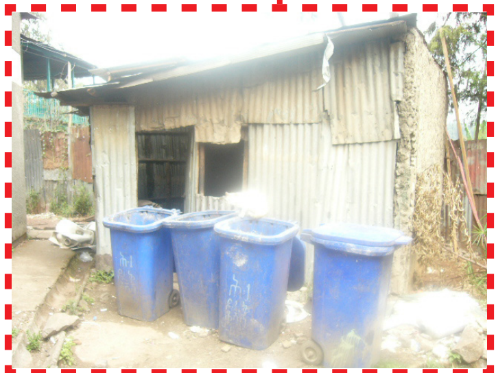
Fig. 7.3 A communal kitchen made from mud and corrugated iron sheet.
