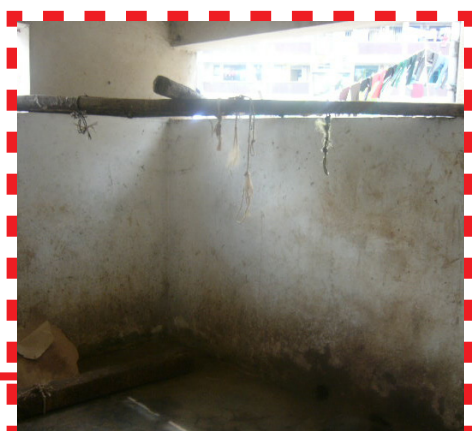
Fig. 7.10 Slaughtering room at ground level of the communal building
