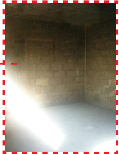
Fig. 6.10 Inside of a slaughtering room of communal building in Gerji
