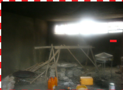
Fig. 8.31 The store serving as Communal kitchen
