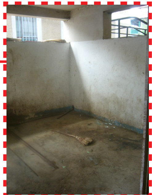
Fig. 7.6 Slaughtering room at ground level of the communal building
