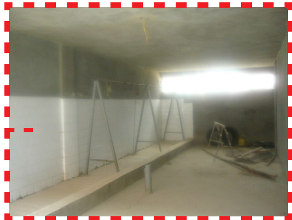
Fig. 8.24 Inside the slaughtering room. ( Metal structure is standing along the slaughtering space for hanging slaughtered livestockes)
