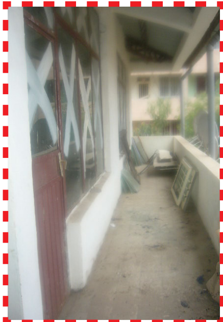
Fig. 8.12 The first floor hall is locked and currently not functional but with the intention of using it for community assembly
