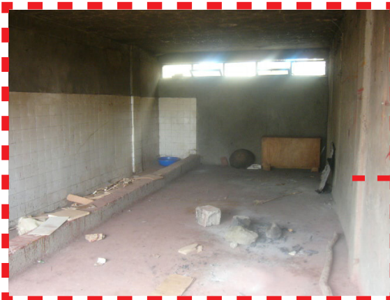
Fig. 8.4 Inside of a Slaughtering room in parcel 01. (The intended slaughtering room is not currently functional and residents use the space as common kitchen and store)
