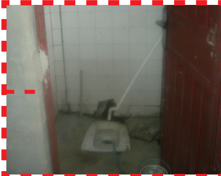
Fig. 8.30 Communal toilet for guards
