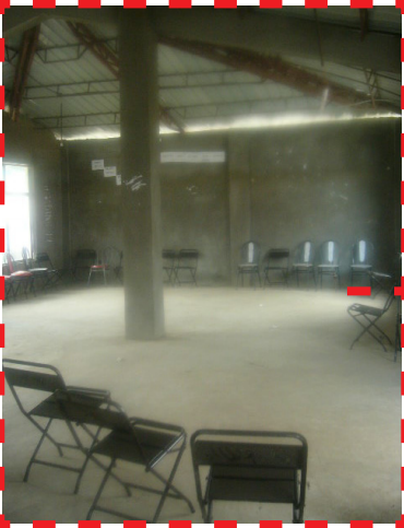
Fig. 8.34 The multi-purpose hall at upper floor.
