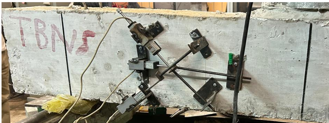
Fig. 5-8 Left Front side of TBNS specimens After failure
