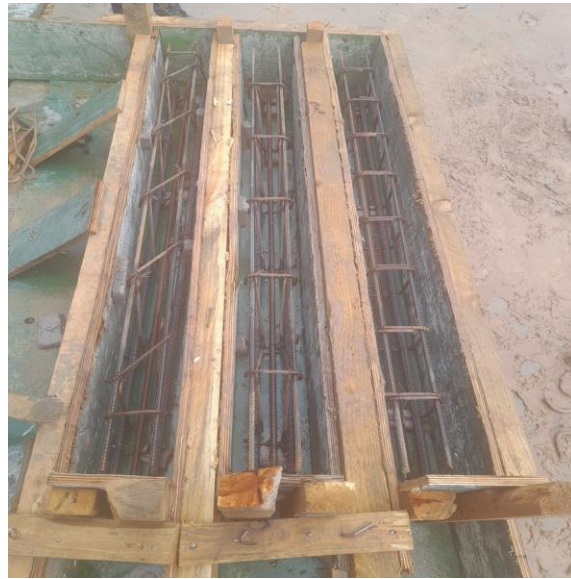
Fig. 3-10 Reinforcement cages set in to formwork
