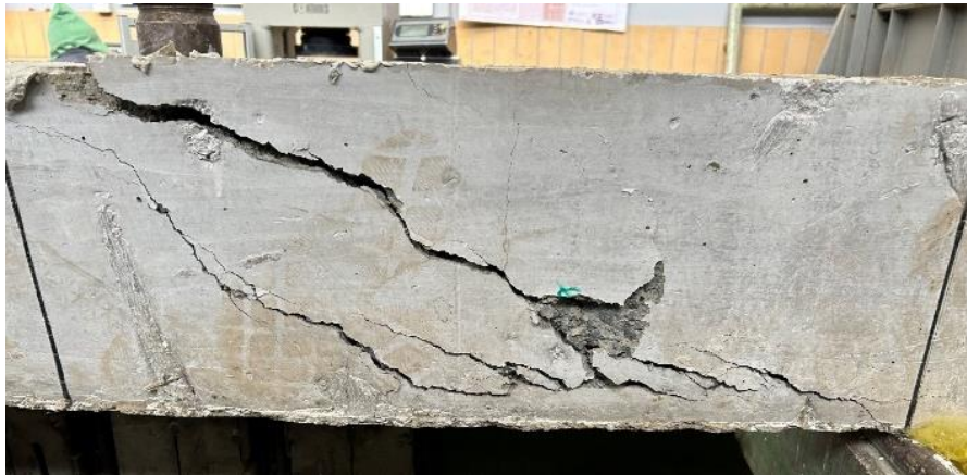
Fig. 5-14 Right Front side of TBS specimens After failure
