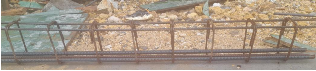
Fig. 3-4 Conventional beam reinforcement cage
