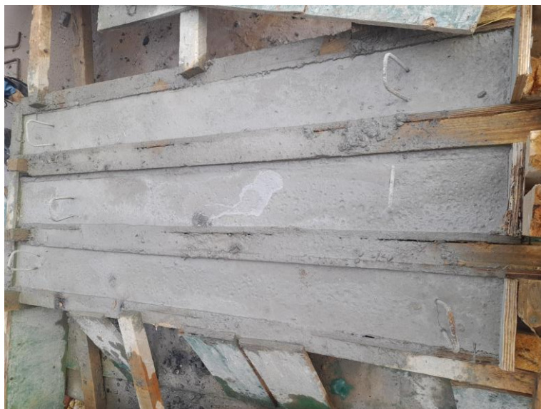
Fig. 3-11 Beam Concrete Casting
