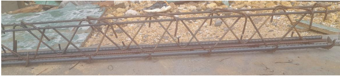
Fig. 3-8 Staggered truss reinforcement cage
