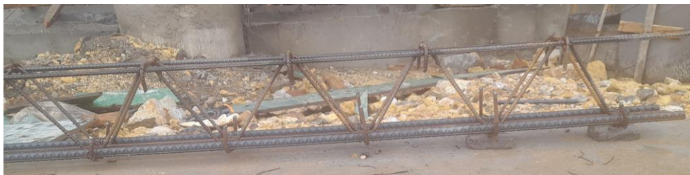
Fig. 3-6 Non-staggered truss reinforcement cage
