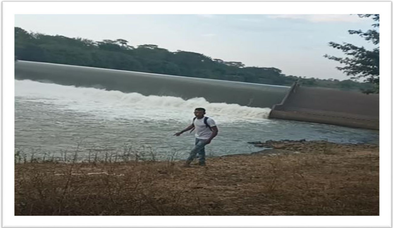
Figure 3. 8. Little Beles Dam 1243 (Diga Dam)
