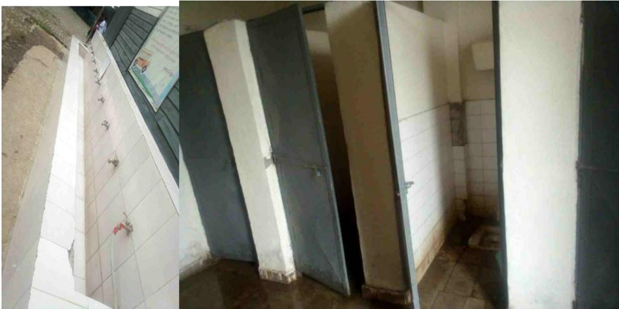
Figure 6: WASH facility inside public schools Source: Author
