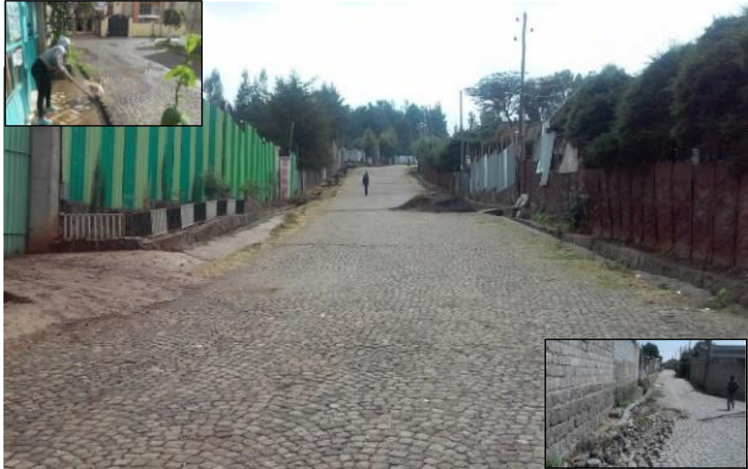
Figure 4: The case site, a typical cobblestone street found in residential areas of Addis Ababa.
