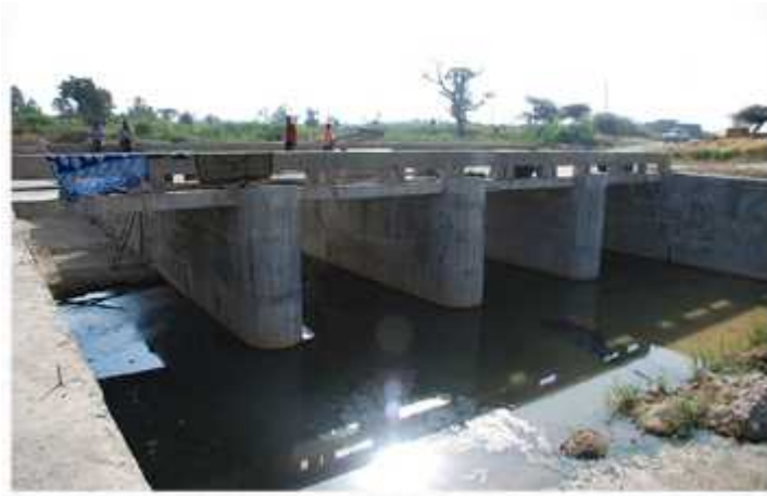
Fig 3.3: The newly-constructed Bulbula River Dam
