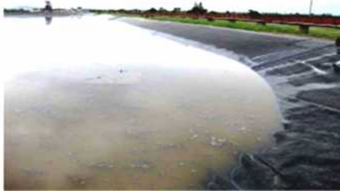
Fig. 5.3: One of the evaporation ponds of Abijata-Shalla Soda Ash Factory.
