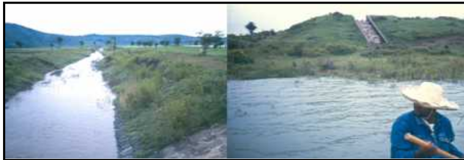
Fig. 1.16: Lake Hora-Kilole after 1989 as water from River Mojo enters lake through the diversion canal. Left: as seen from the canal and right: as seen from lake water surface or from boat.
